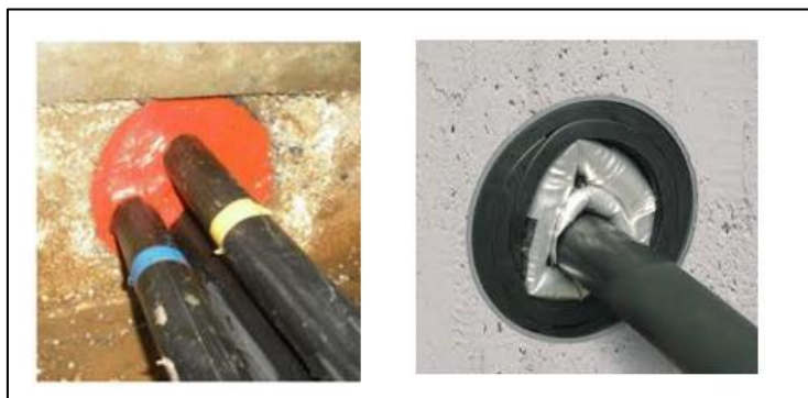
Figure 8: Rayflate (Right) and Nofirno (Left) Cable Duct Sealing Systems
