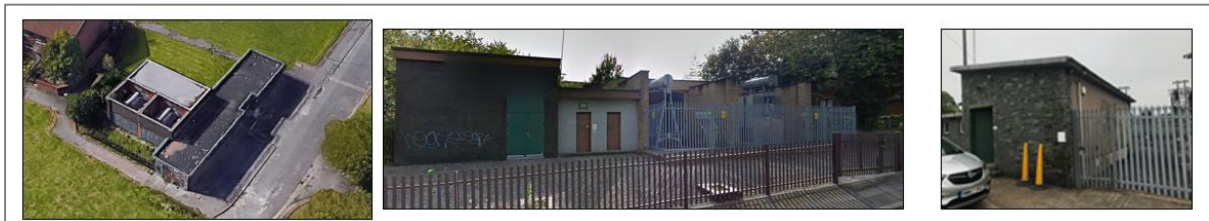
Figure 26: Archetypal Substations Selected for Case Studies (From left to right Pendleton, Southeast Macclesfield & Windermere)
