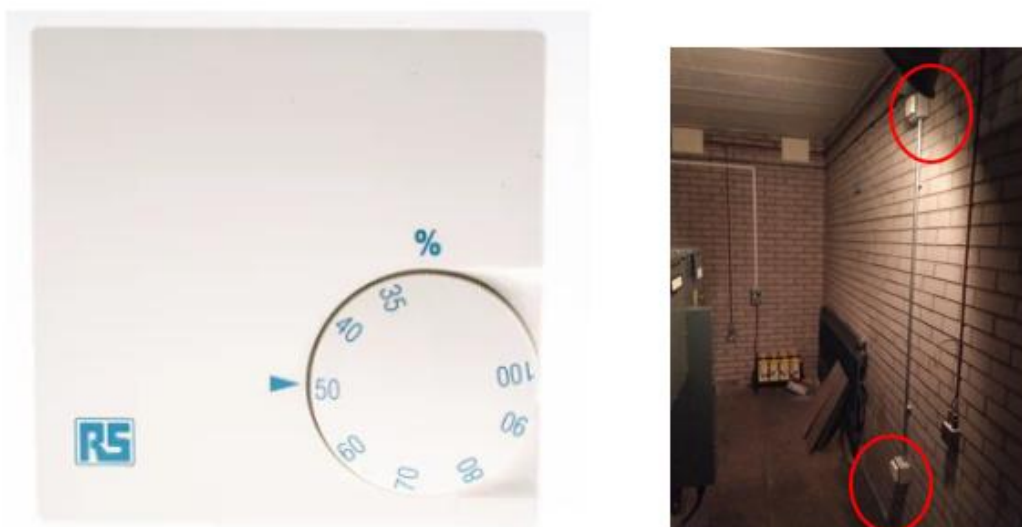
Figure 39: Enhanced Dehumidification Controls:
