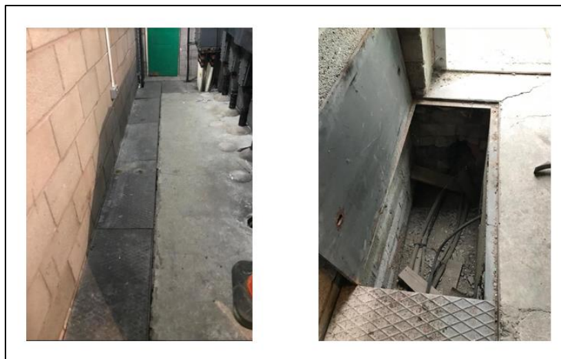
Figure 3: Pendleton Primary Cable Trenches
