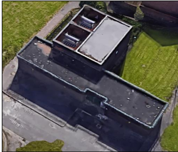
Figure 2: Aerial View of Pendleton Primary Substation
