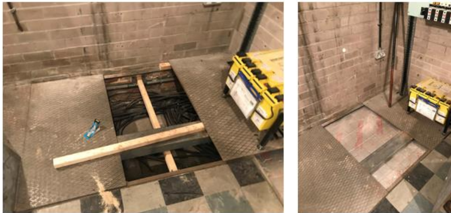
Figure 43: Trench Splitter System in Construction and Installed
