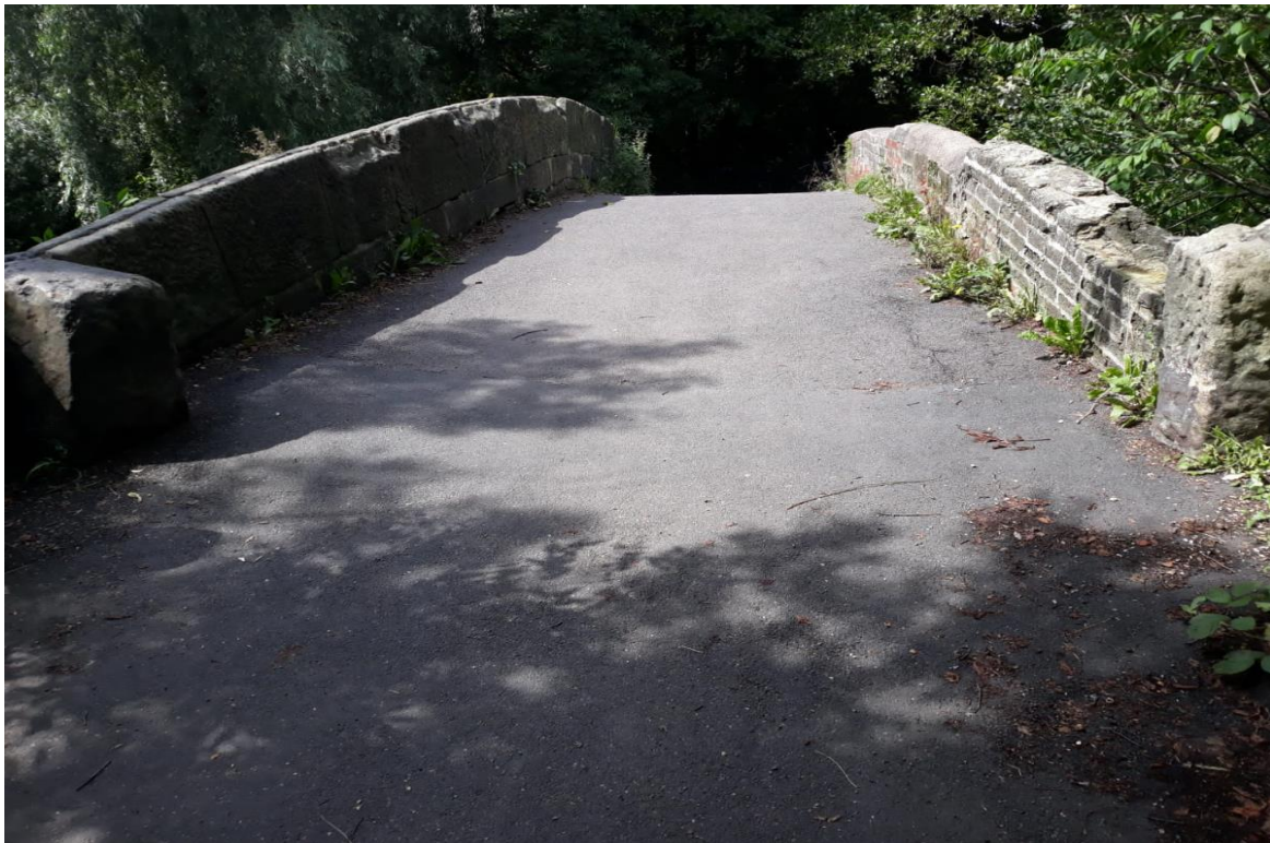
Figure 5.14 Wrigley Head Bridge
