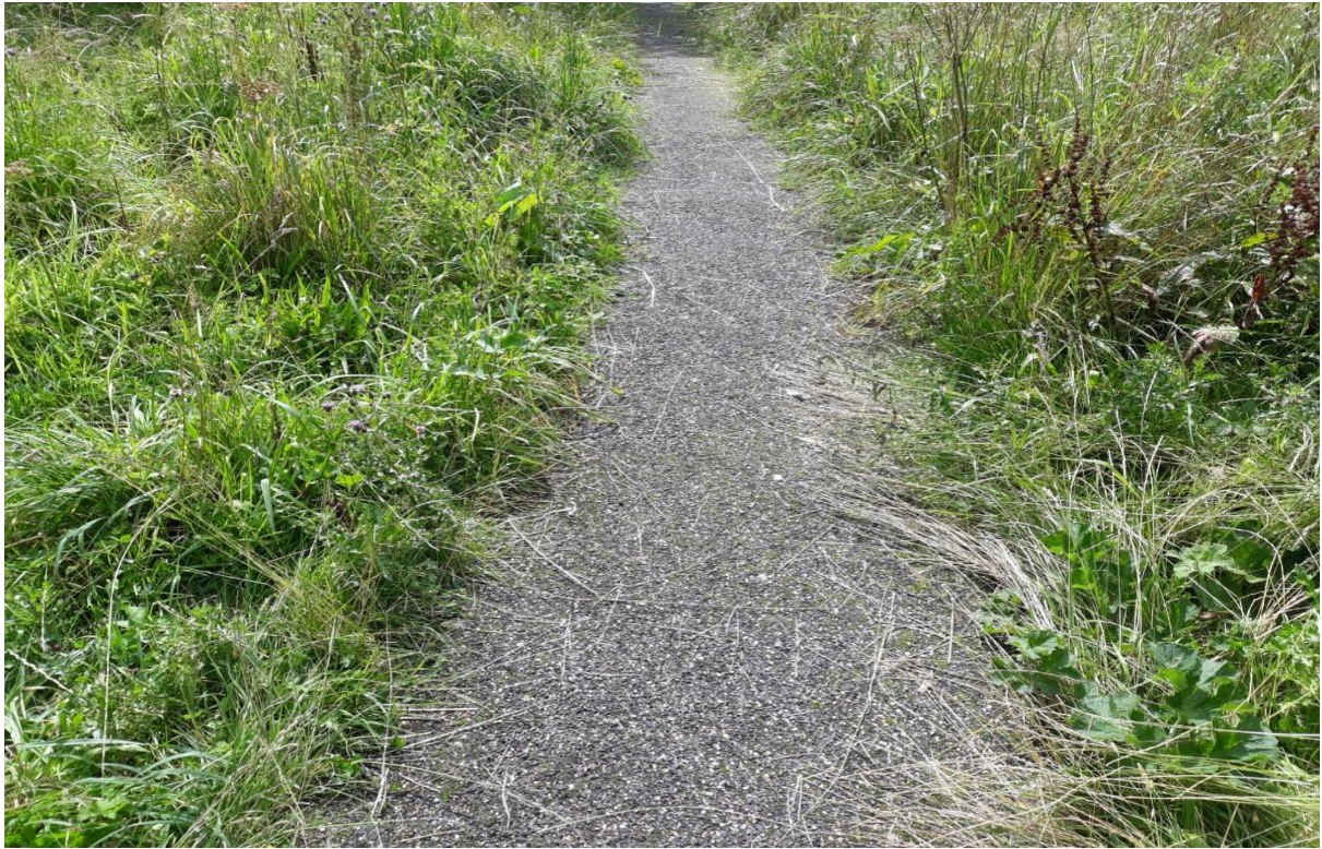
Figure 5.20 Wrigley Head improved footpath
