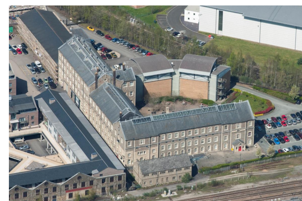
Image 2: Aerial view of HE Swindon site
