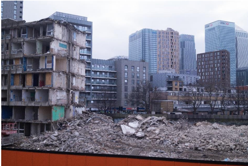
Figure 6: Demolished Robin Hood Estates, East London, 2018
