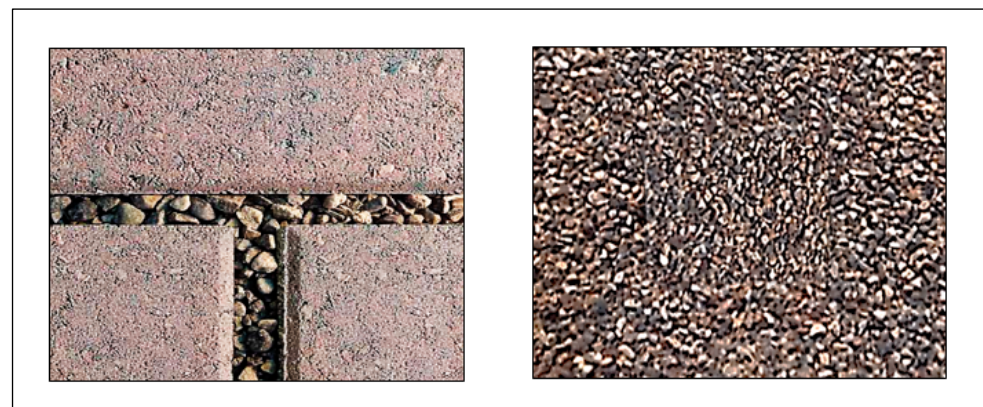
Figure 11. PICP joints’ filling.
