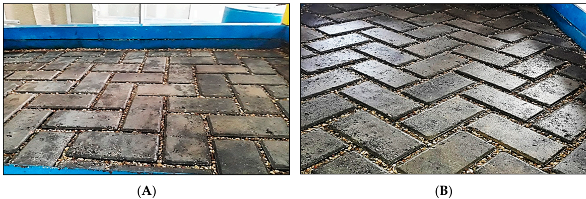
Figure 16. PICP’s surface patterns. (A) 90° herringbone; (B) 45° herringbone.
