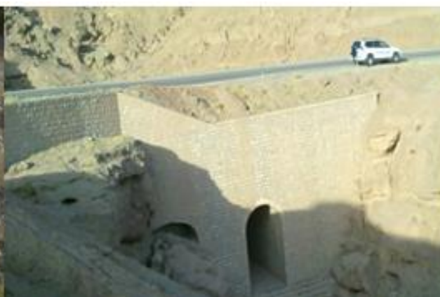
Fig. 17. Example of a bridge by an innovative method.
