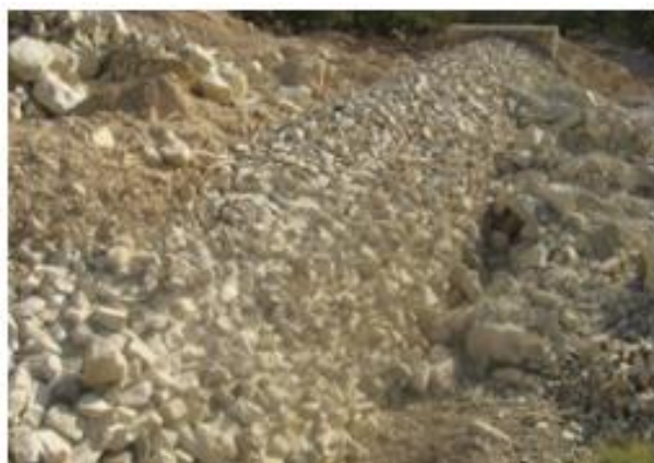
Fig. 16. A combined embankment.
