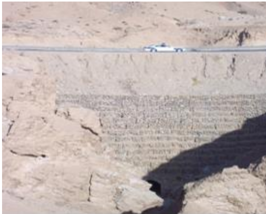
Fig 1. Overview of the bridge.
