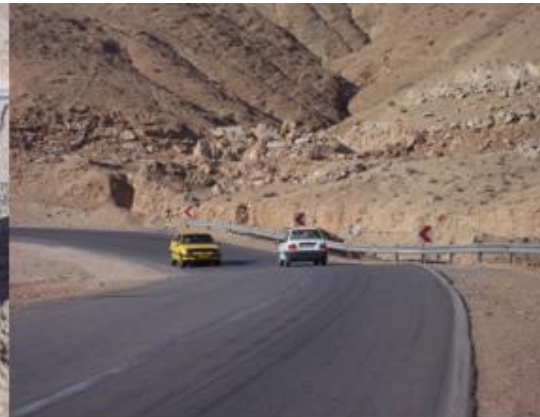
Fig 2. Settlement created at the location of the bridge.
