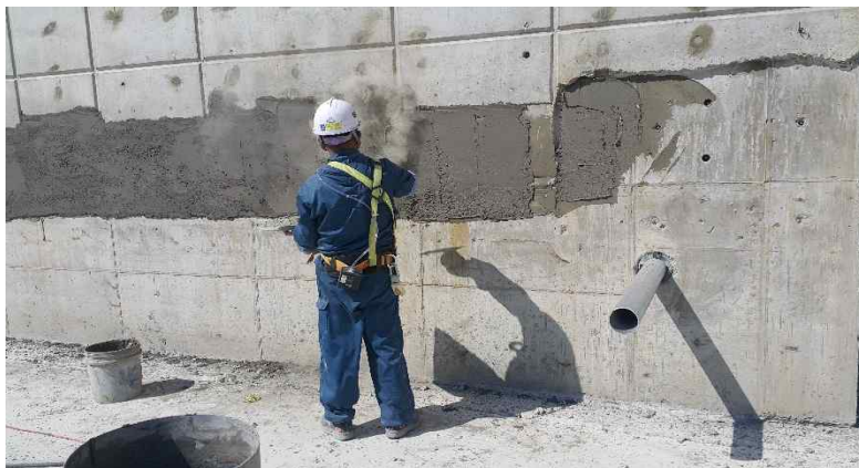
Figure 3-1. Concrete chipping(a), grinding(b) and plastering(c) work
