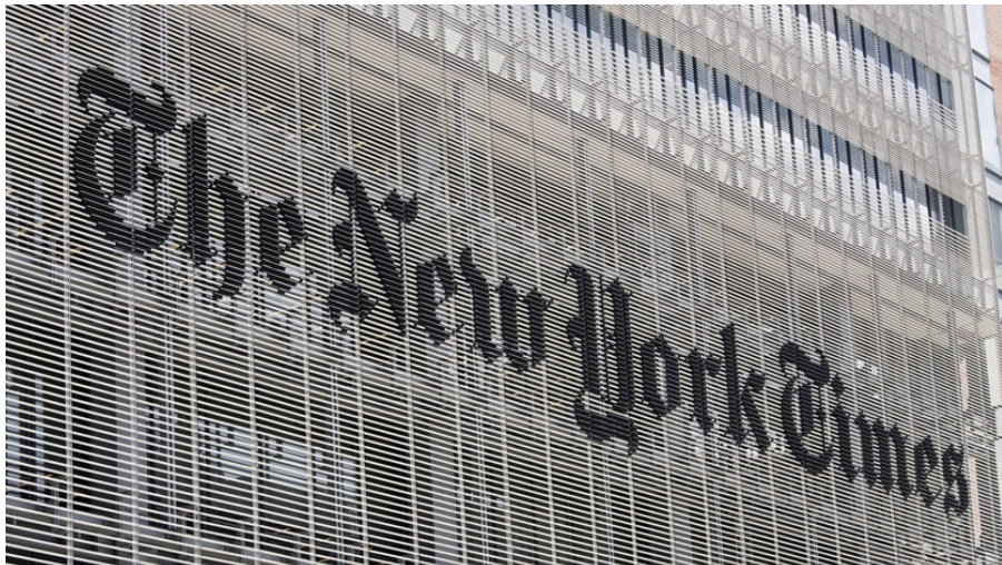
Figure 2-8. The New York Times Building Facade
