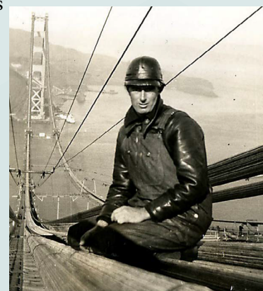
A Golden Gate construction worker wears a Bullard “hard boiled hat” in this photograph, circa 1936. Credit: Labor Archives and Research Center, J. Paul Leonard Library, San Francisco State University
