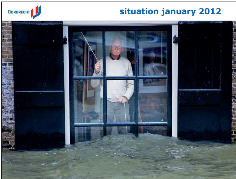
Figure 8.4: Flood-proof window in Dordrecht
