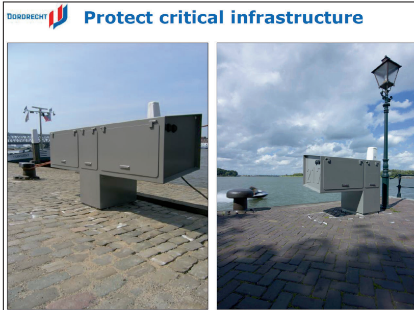
Figure 8.7: Elevated critical infrastructure
