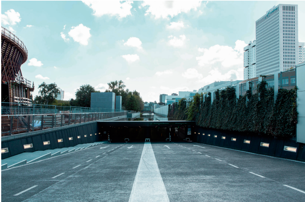
Figure 7.4: Museumplein parking garage
