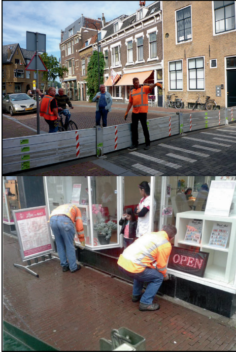
Figure 8.8: Placement of flood barriers on the streets and in front of shops during the vloedschotten exercise
