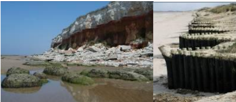
Erosion at Hunstanton Cliffs (left) and erosion defences at Brancaster (right). Both photos supplied by Environment Agency
