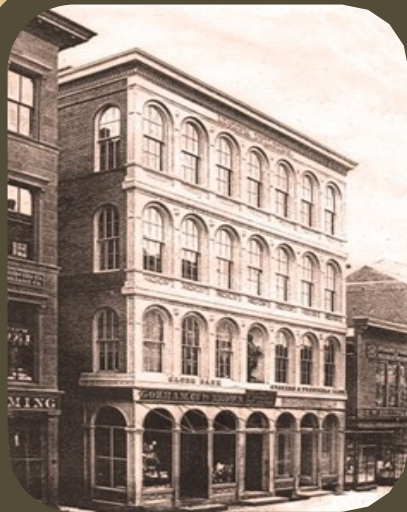
Figure 1 Lyceum Building Photo courtesy of RIHS
