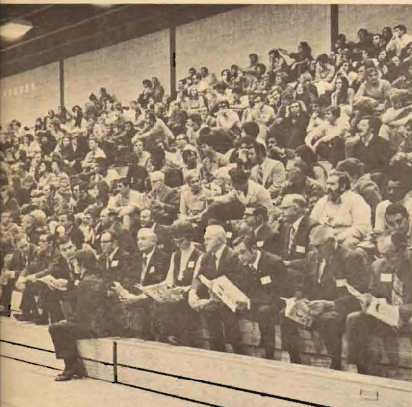
by new gymnasium which holds 2,700 people.
