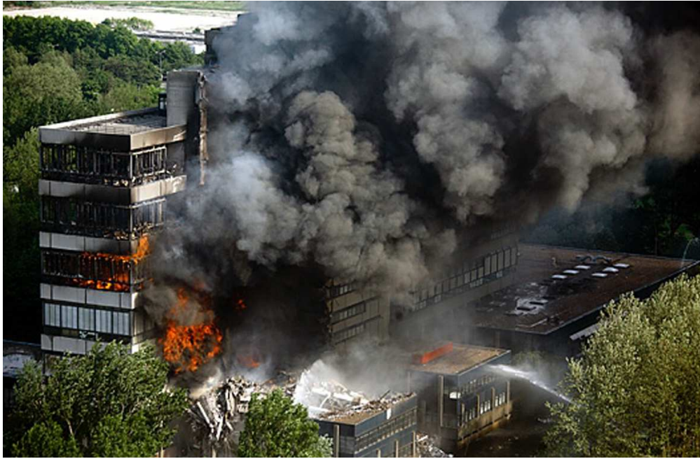
The Faculty of Architecture building being on fire 99x64mm (300 x 300 DPI)
