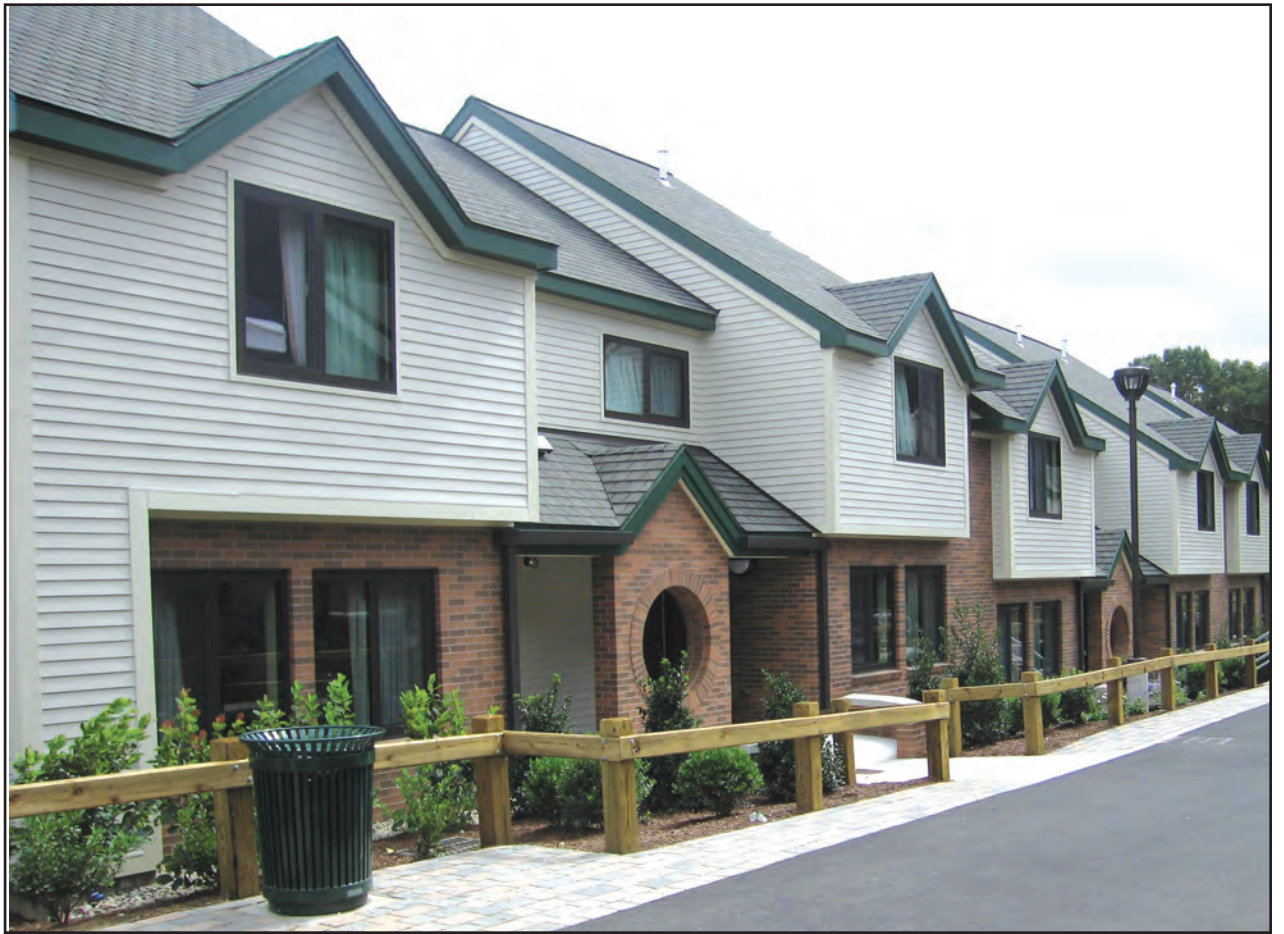
The new O & P townhouse blocks have added nearly 100 extra beds in the living community designed for the senior class. (Ashley McNamara)
