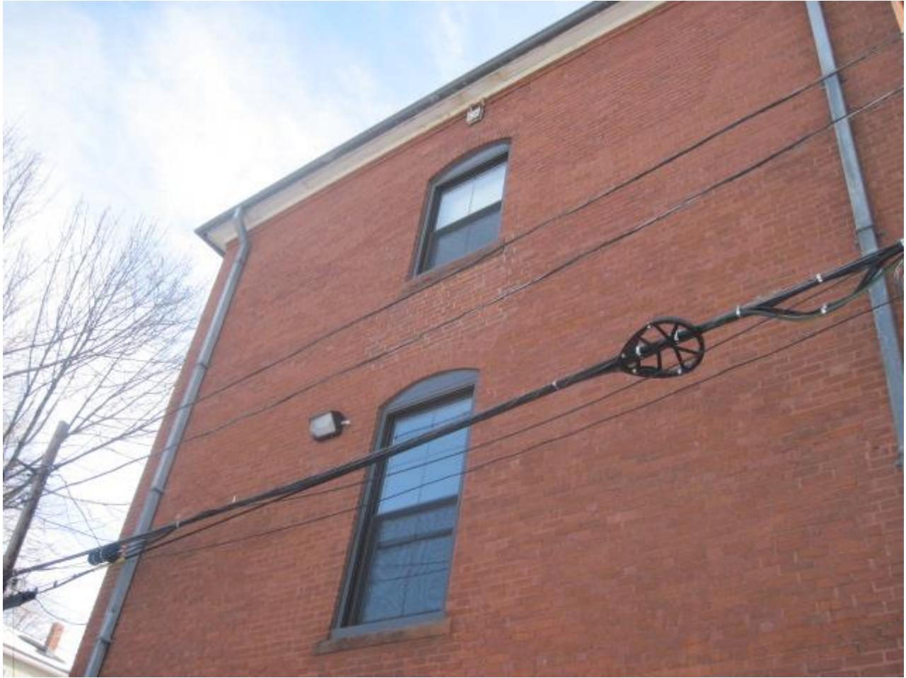
Photograph 22: Openings – Rear First and Second Floor
