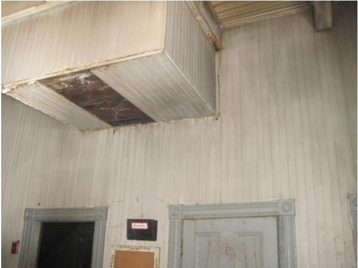
Photograph 35: Interior Features - Walls
