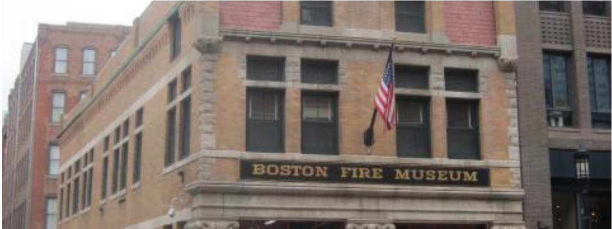
Photograph 12: Trim and Secondary Features - Window Trim
