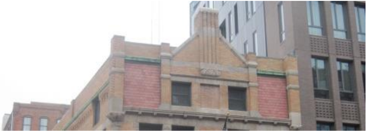
Photograph 13: Trim and Secondary Features – Roof
