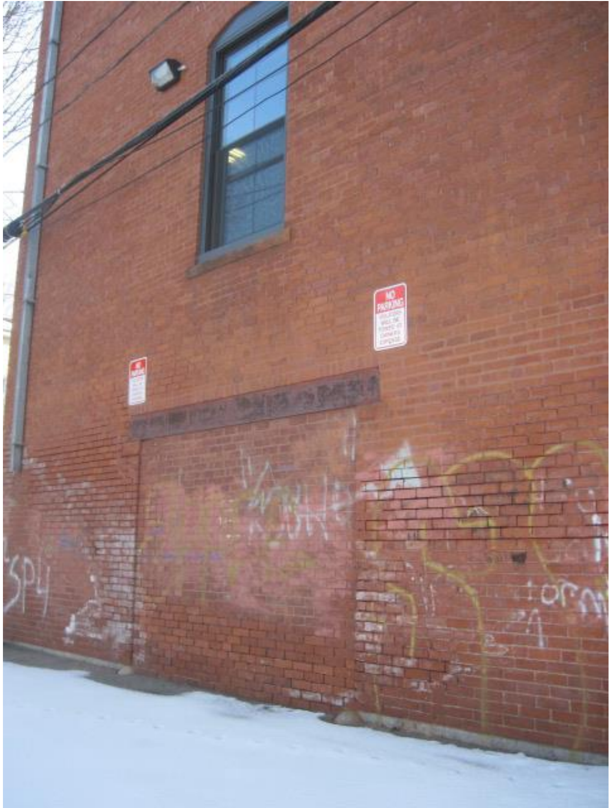
Photograph 23: Openings – Rear – Basement and First Floors
