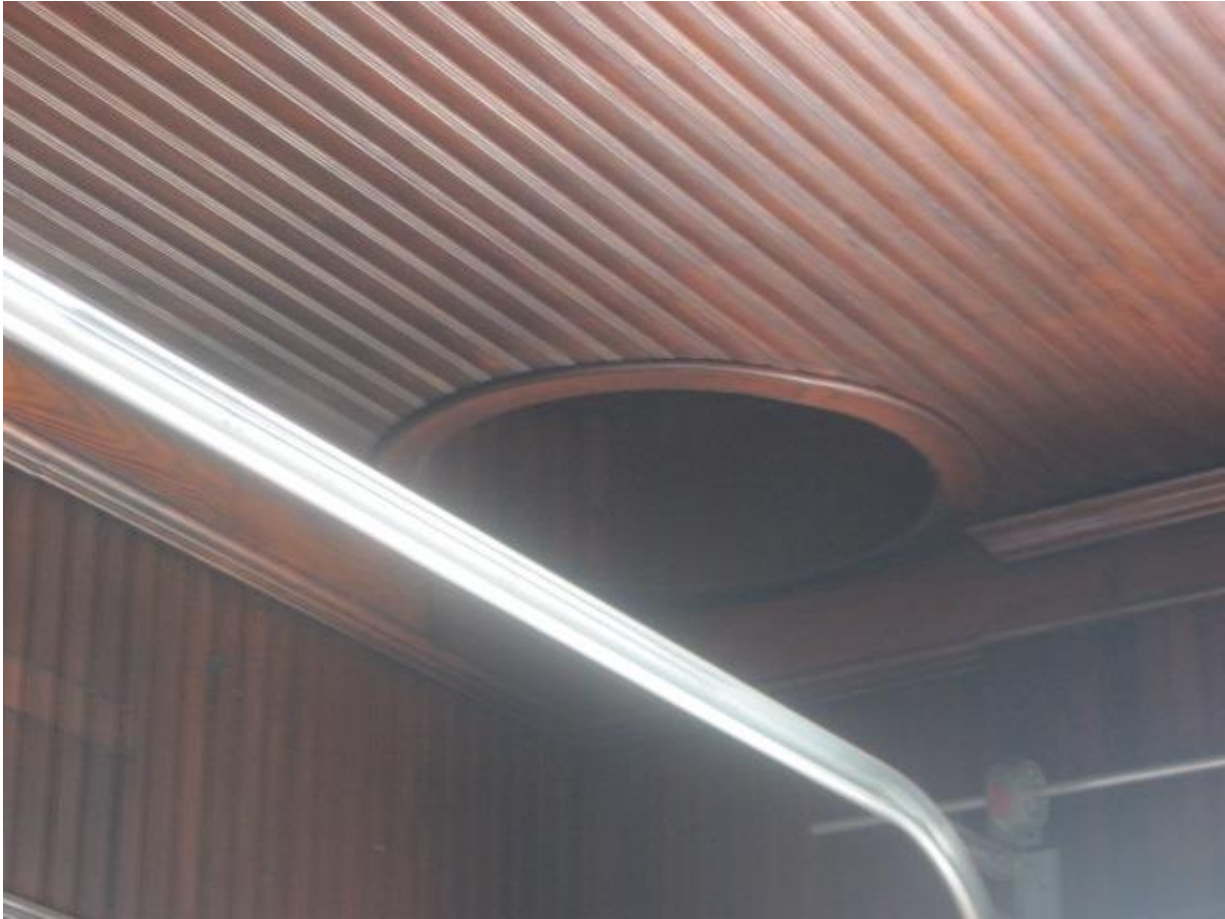
Photograph 56: Trim and Secondary Features – Interior Sliding Pole
