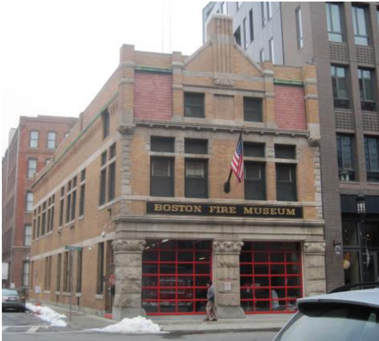
Photograph 11; - Trim and Secondary Features – Piers
