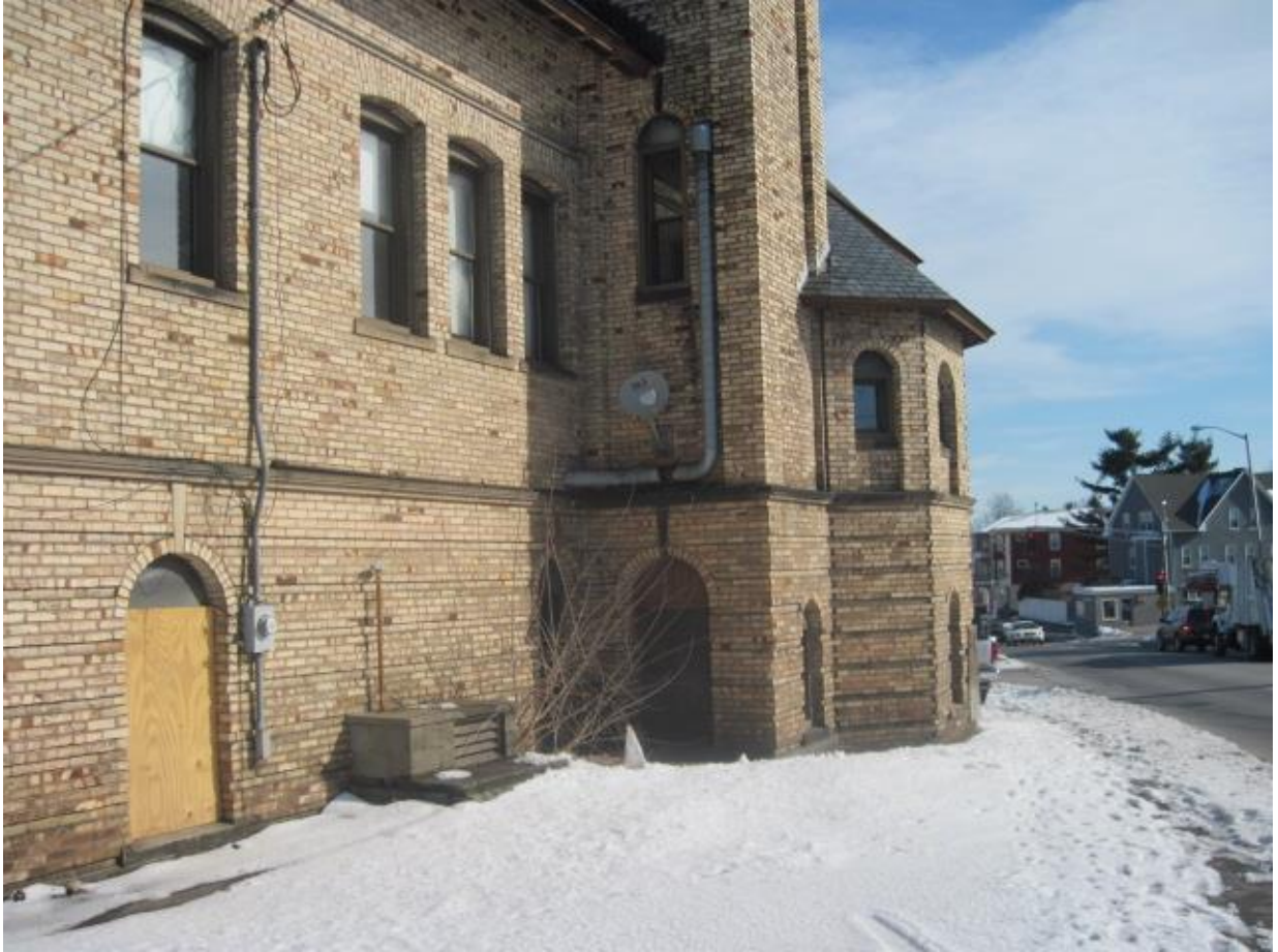
Photograph 43: Window Openings – First Floor
