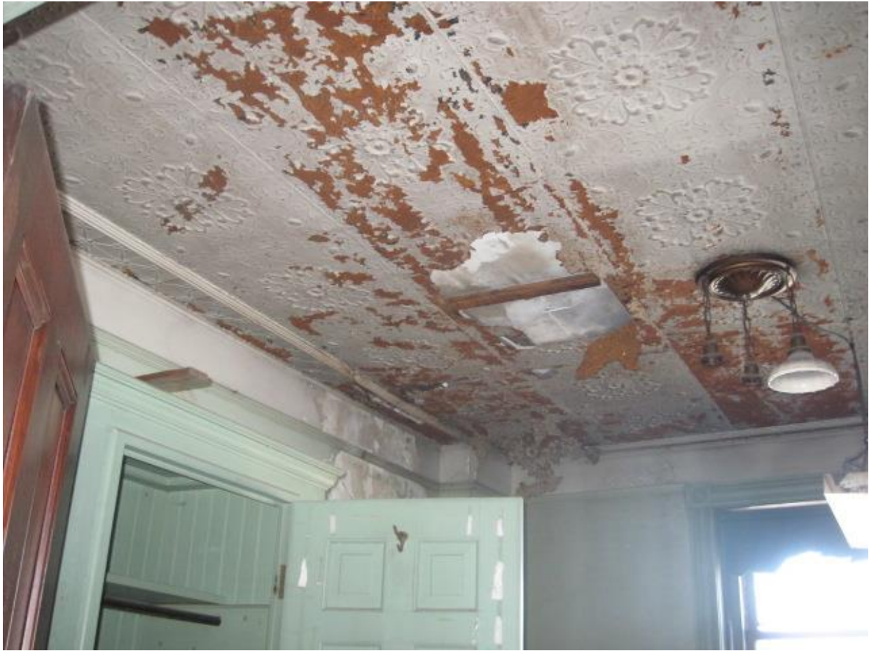
Photograph 38: Finishes and Materials – Second Floor Ceiling
