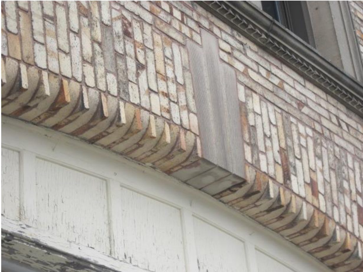
Photograph 49: Craft Details – Brick Arch
