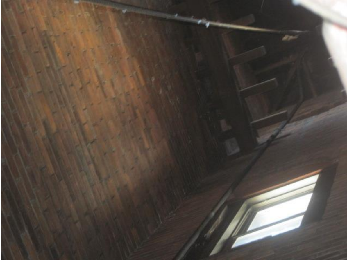
Photograph 57: Trim and Secondary Features – Interior Tower
