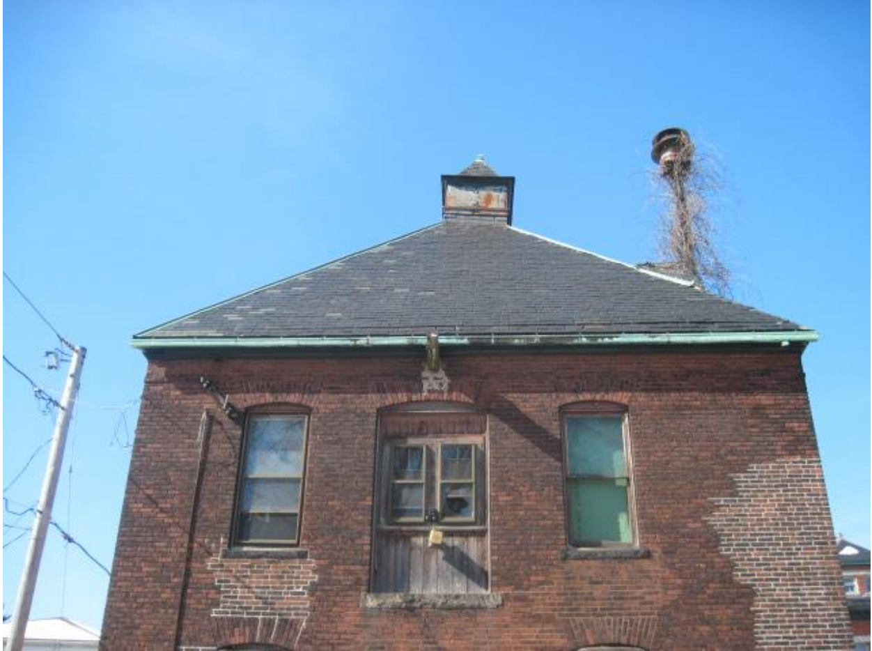
Photograph 29: Roof and Roof Features – Rear
