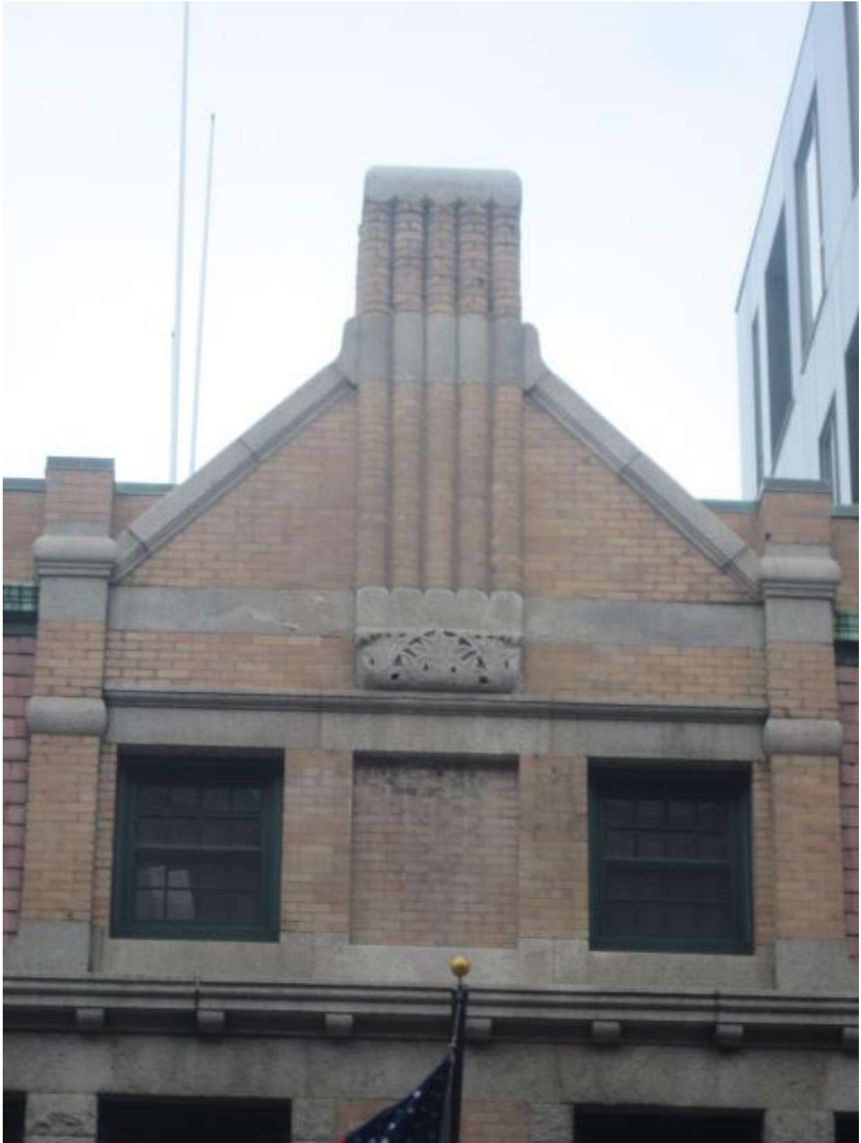
Photograph 8: Window Openings – Front, Third Floor
