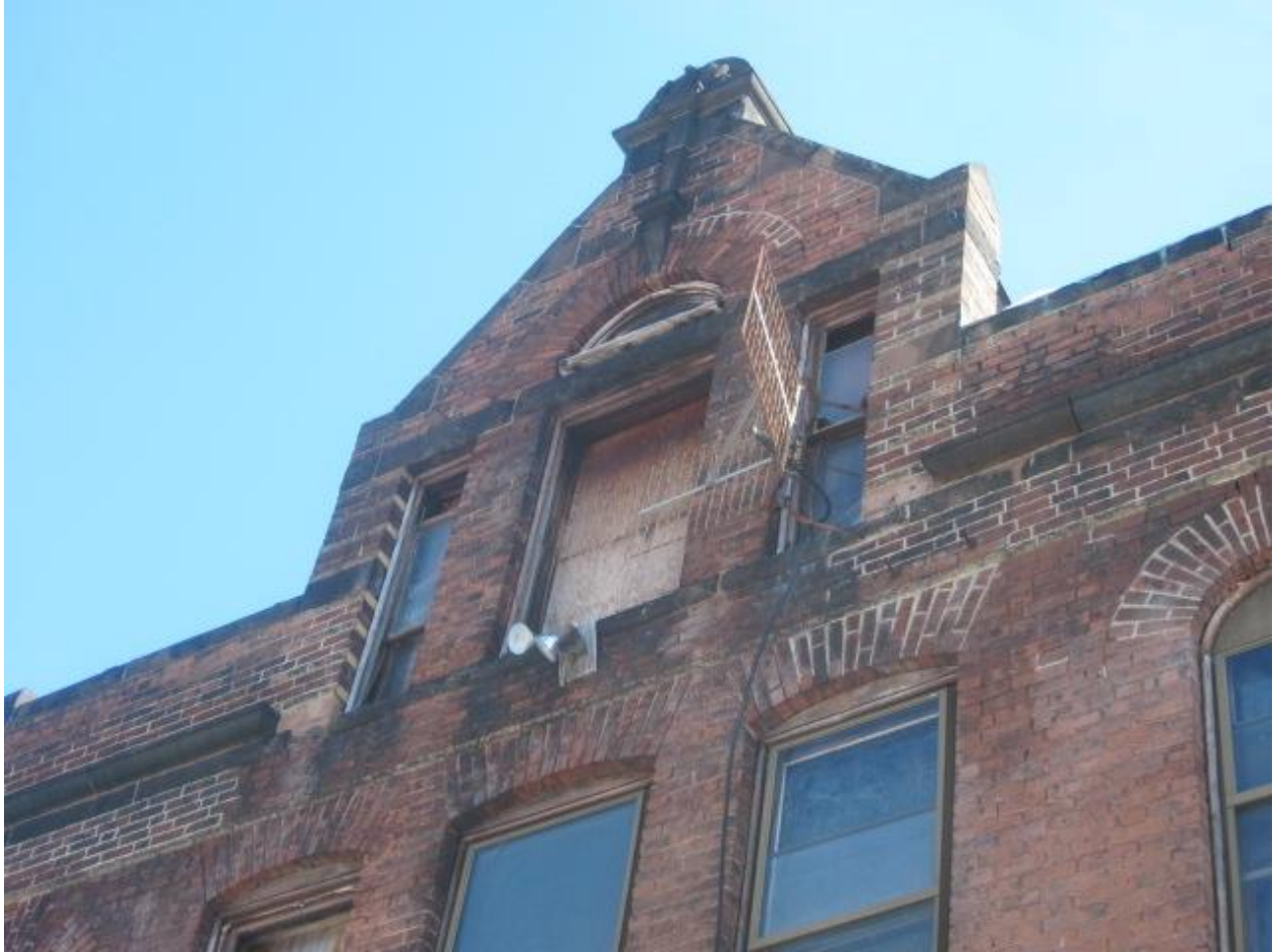
Photograph 30: Roof and Roof Features – Front
