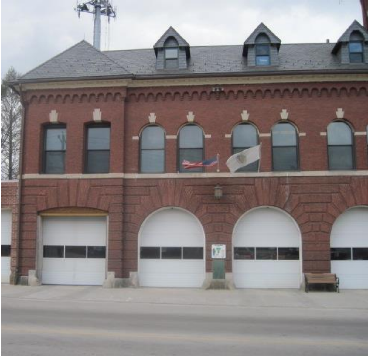
Photograph 60: Trim and Secondary Features – Façade
