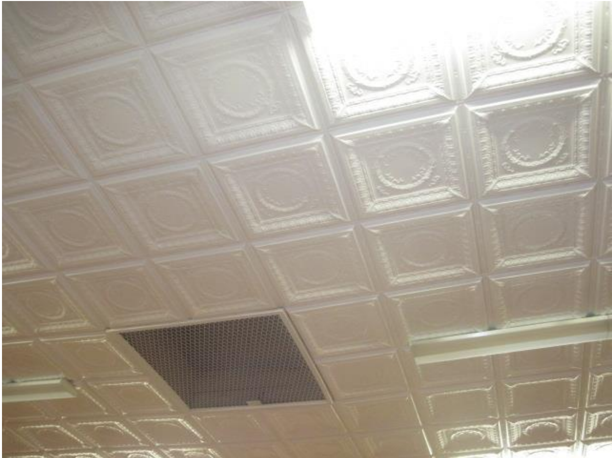
Photograph 64: Interior Finishes - Ceiling
