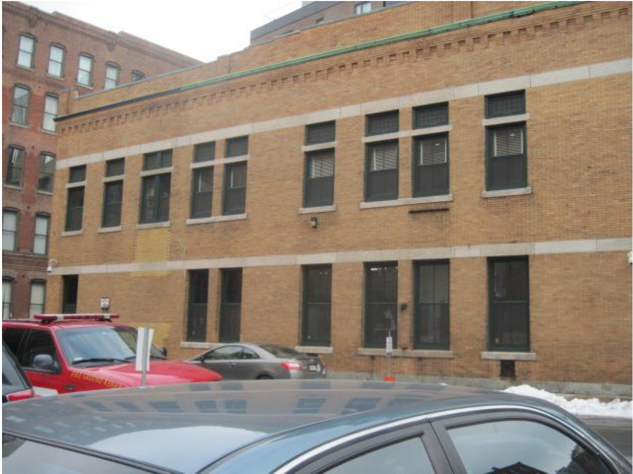
Photograph 9: Window Openings – Side, First and Second Floors
