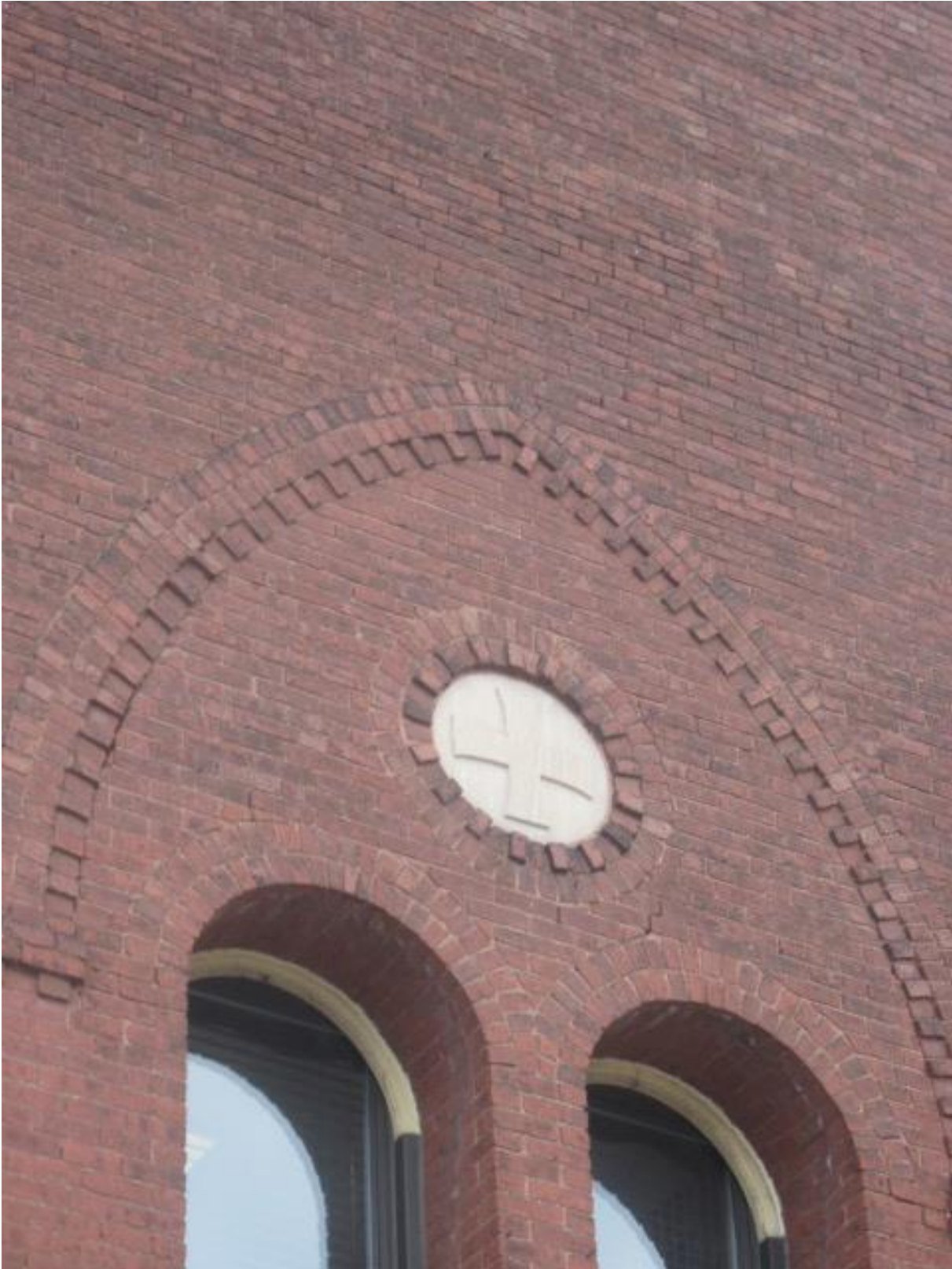
Photograph 68: Trim and Secondary Features – Maltese Cross
