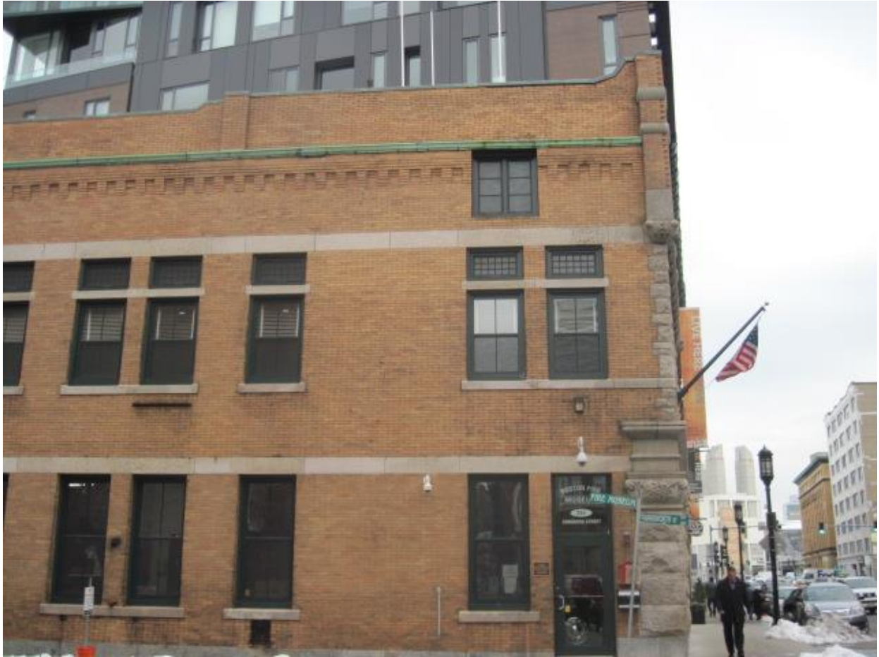
Photograph 10: Window Openings – Side
