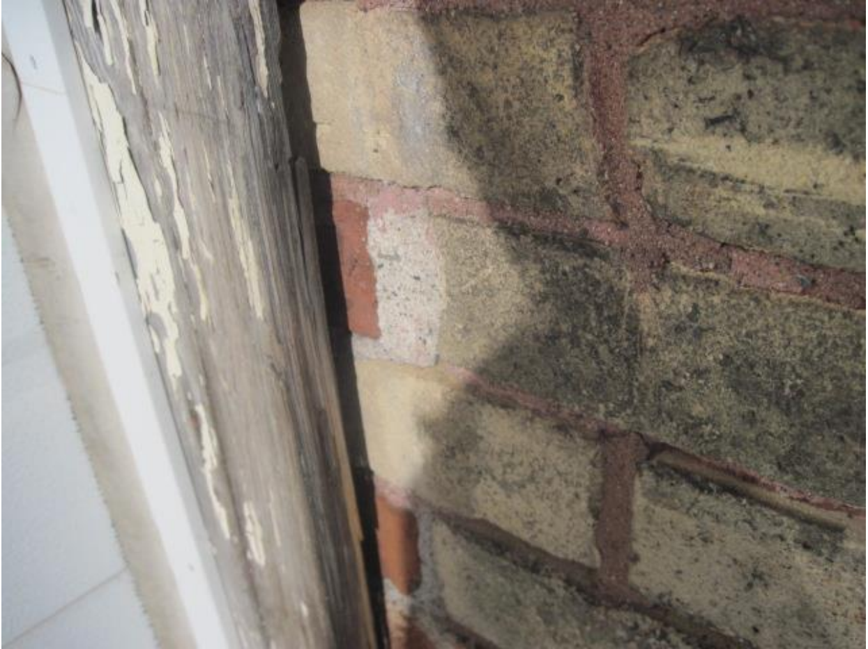
Photograph 48: Materials – Red and Yellow Brick
