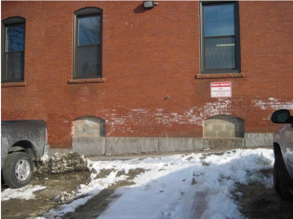
Photograph 21: Window Openings – Side, Basement
