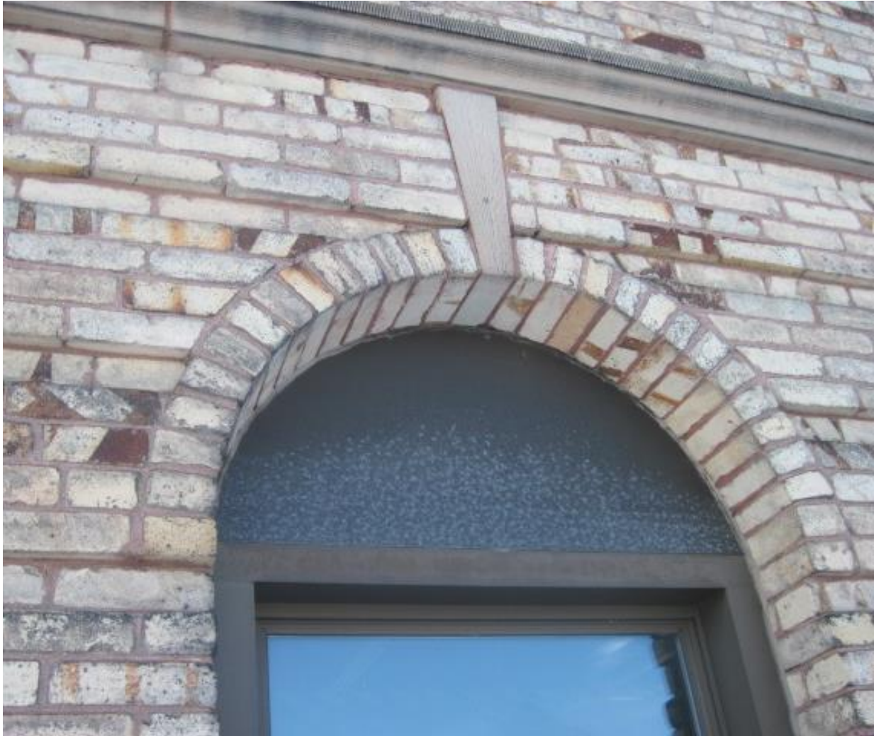
Photograph 47: Trim and Secondary Features – Arched Windows
