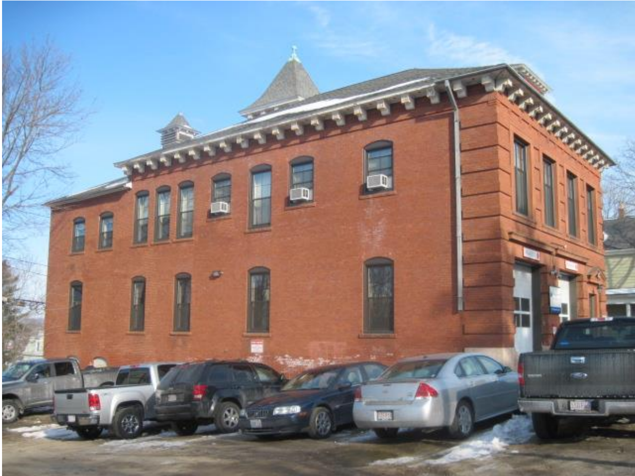
Photograph 20: Window Openings – Side
