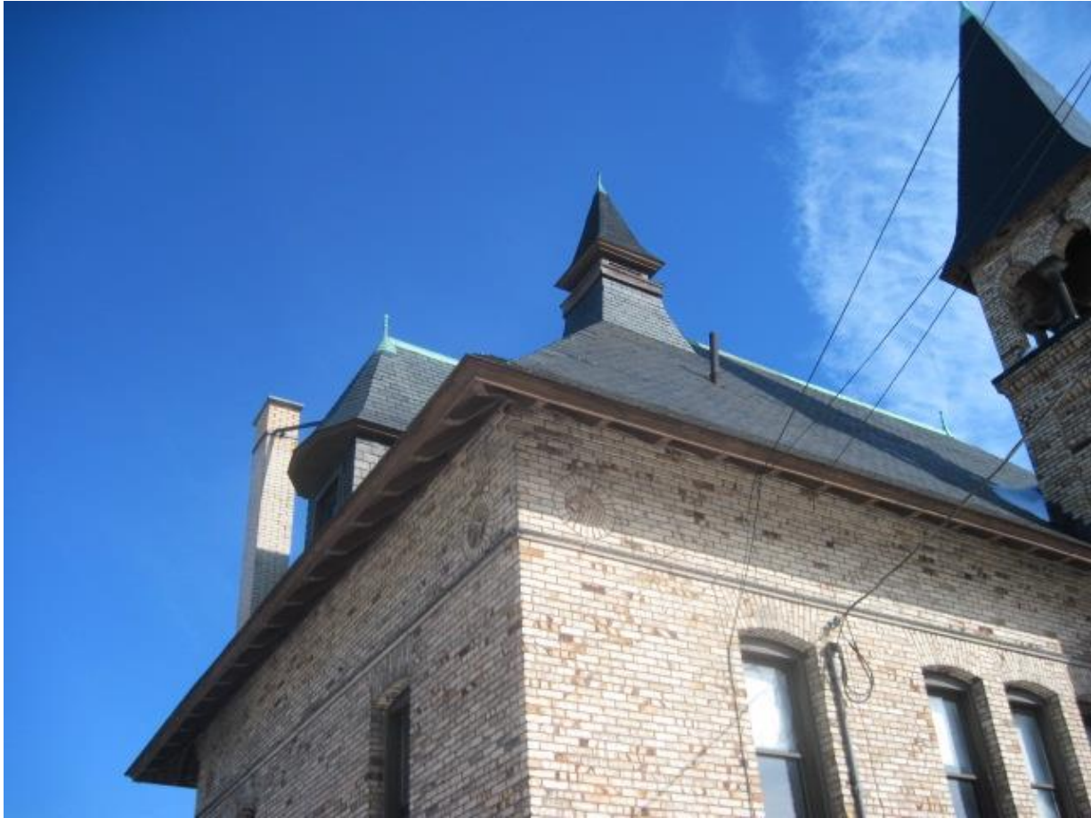
Photograph 42: Roof and Roof Features
