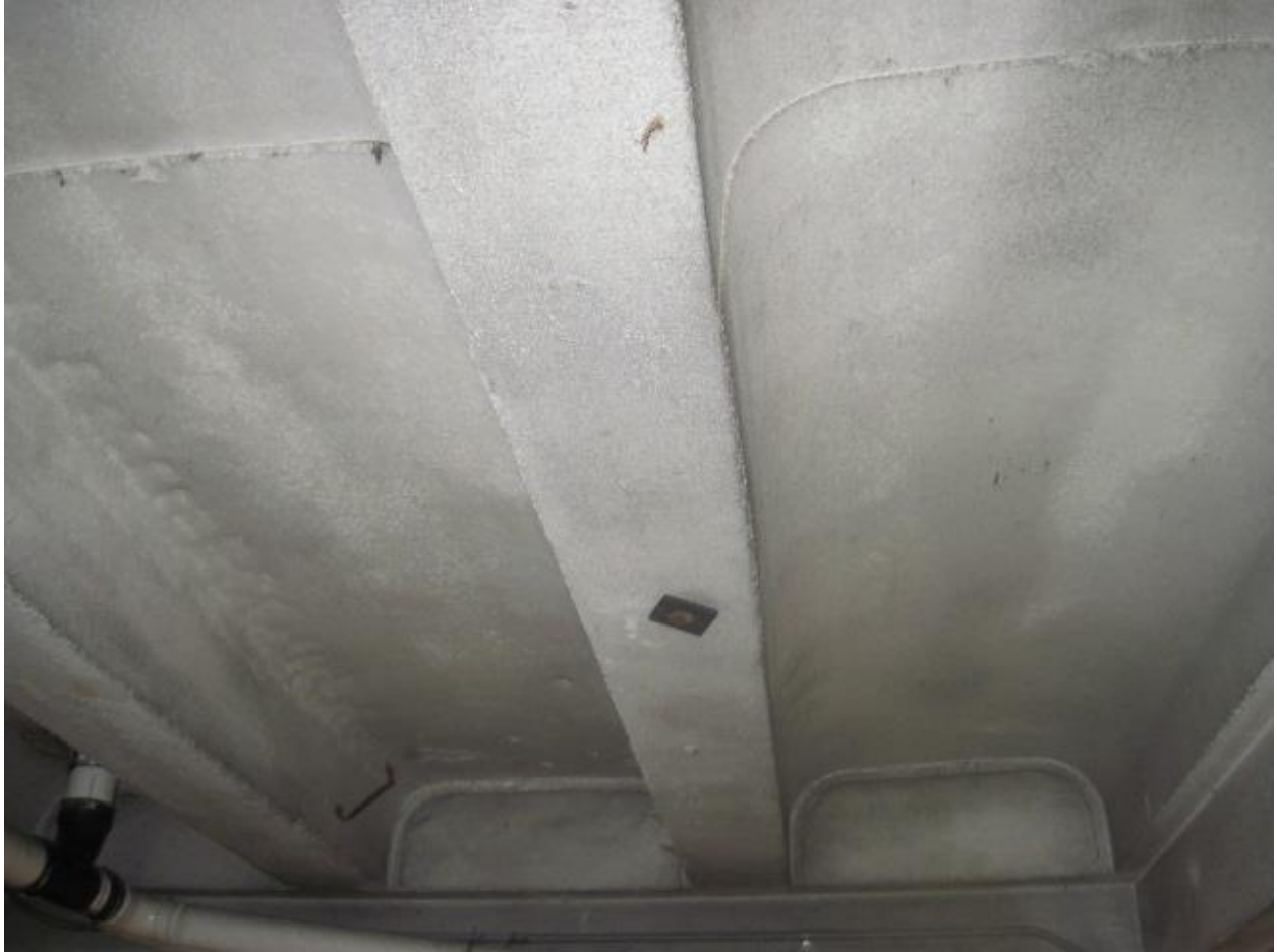
Photograph 65: Exposed Structure – Interior
