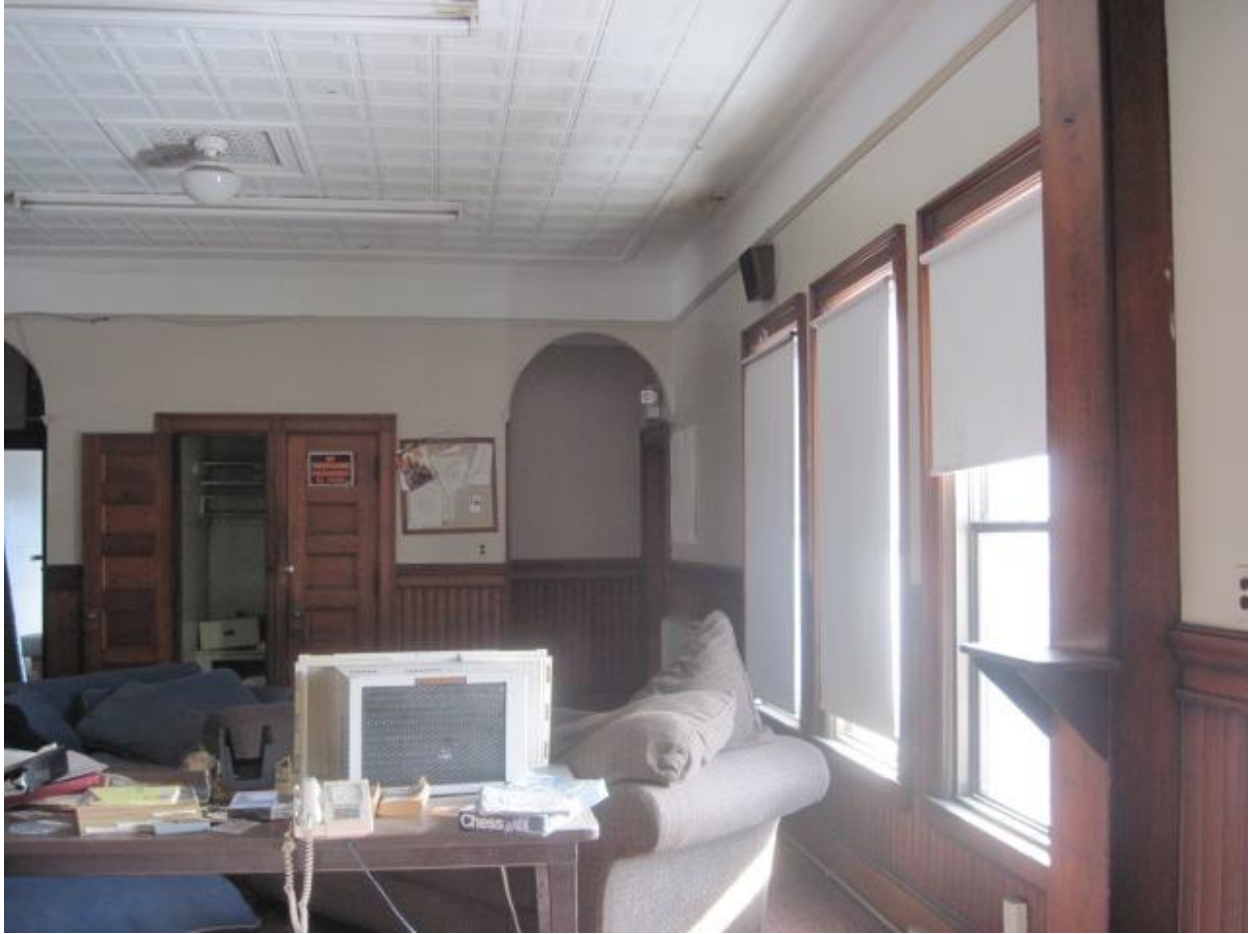
Photograph 54: Finishes and Materials - Ceiling
