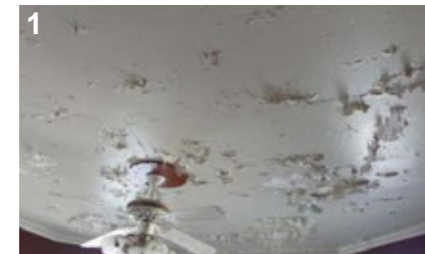
1. Interior bedroom ceiling
