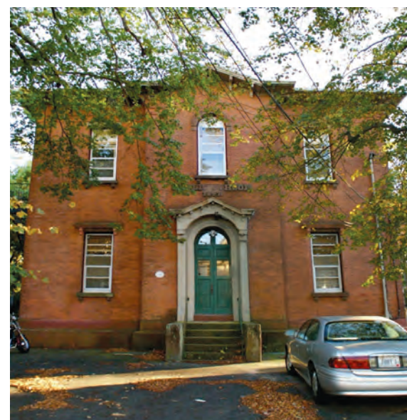
Brick Masonry Walls
