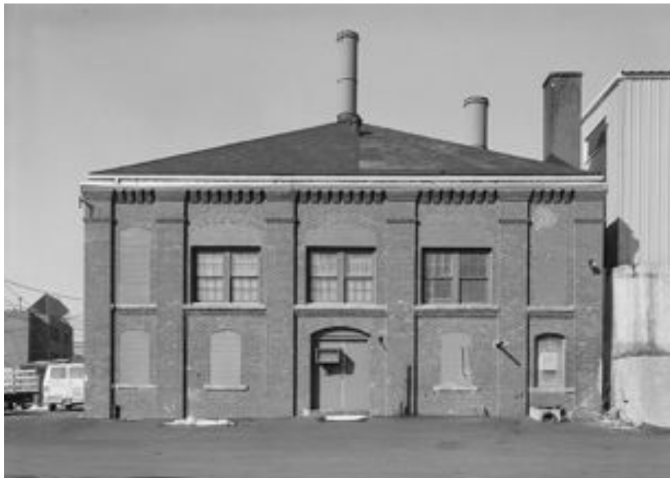
Sludge Press House at the Fields Point Wastewater Treatment Facility, March 1989. This building no longer exists. National Park Service
