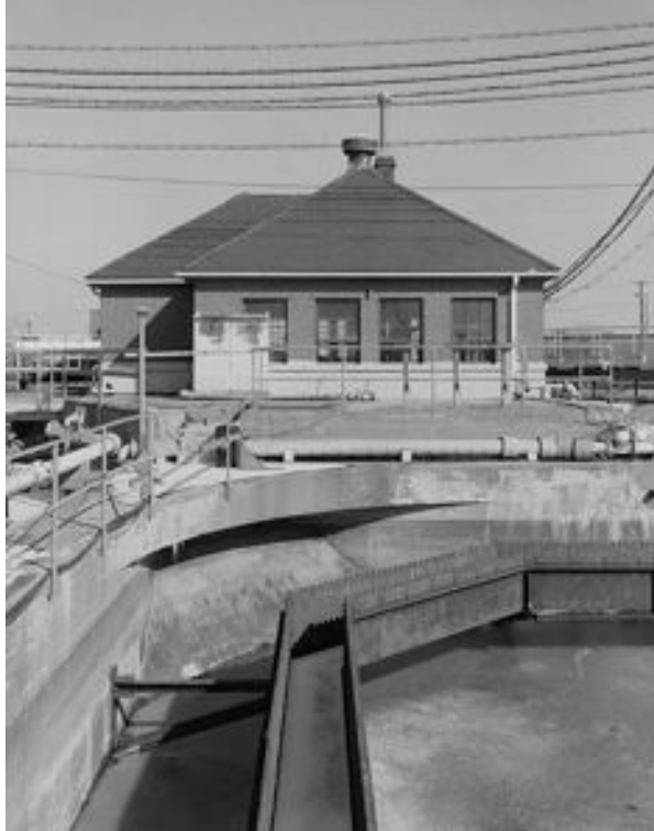
Return Sludge Pumping Station at the Fields Point Wastewater Treatment Facility, March 1989. Constructed in 1934, this accompanies the Chemical House as the only two buildings left from the original facility. National Park Service .
