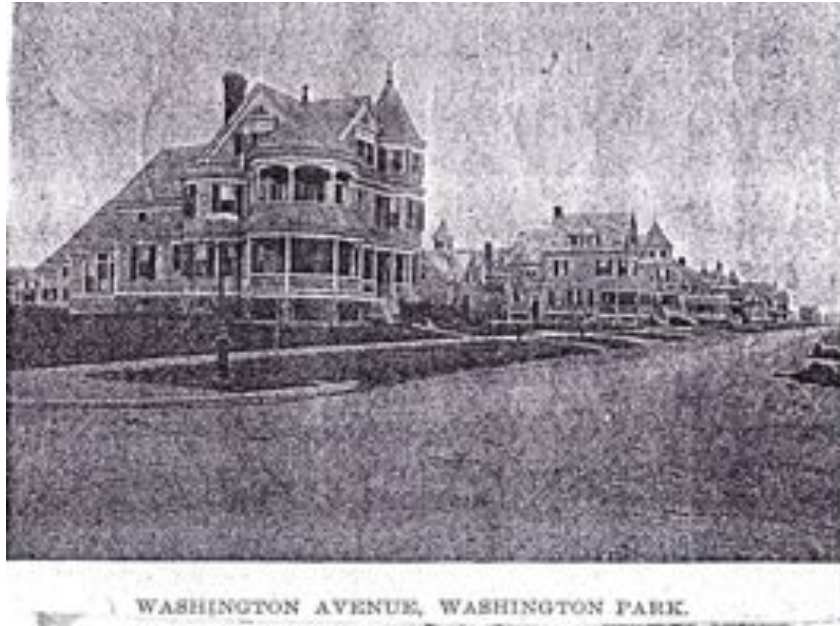
View of 305 Washington Avenue, looking northeast. The two-story porch on the southwest corner is no longer extant, but the three-story turret on the southeast corner still remains. Note 287 Washington Avenue in the background. Rhode Island Historical Society.
