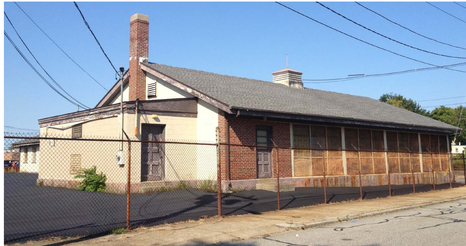
Current building at 945 Eddy Street.
