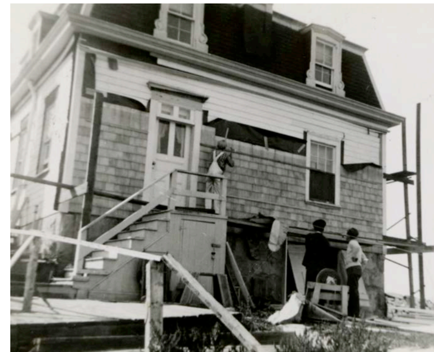
Pomham Rocks was sheathed in shingles and underwent restoration in 1939 under lighthouse keeper William J. Howard.
