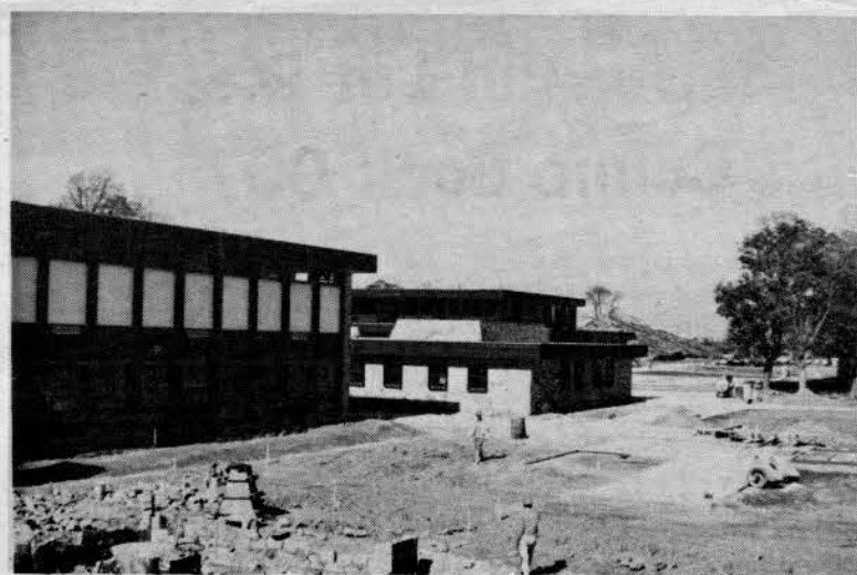
Bristol Campus under construction.
