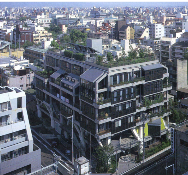
View _main corner view
