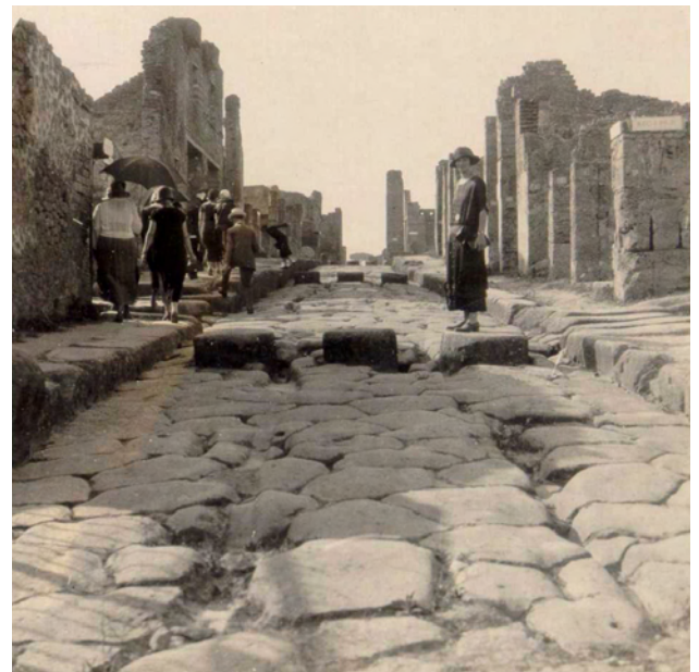
Integrated Design _ road, water & steps
