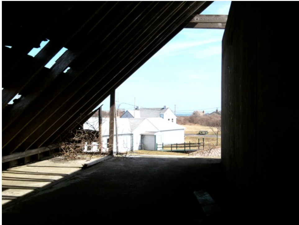
[Fig. 26] View of the west elevation of Room 2-2, looking east.
