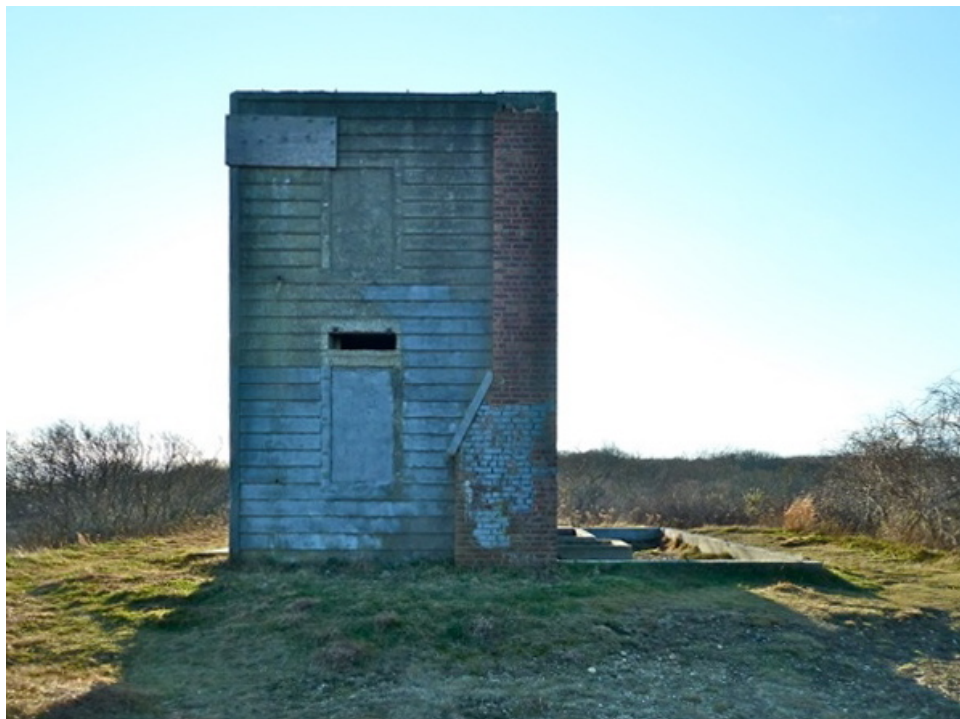
[Fig. 6] East elevation, looking west.
