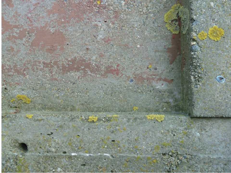
[Fig. 24] Detail of blind window on the north elevation. Note the plastic screw anchor for a wooden jamb, reddish-brown paint in blind window, and trace of white paint on the concrete area formed to mimic simple drop wooden board.
