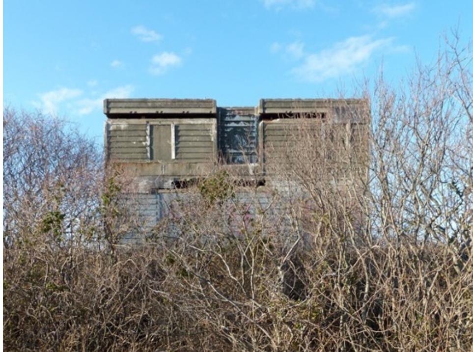
[Fig. 3] South elevation, looking north.
