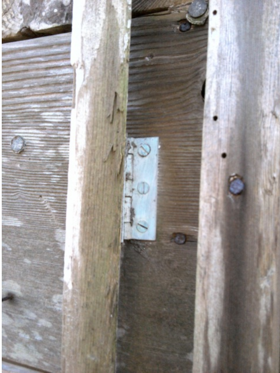
[Fig. 23] Detail of ribbon window sash remnant. Note original hinge and screws, all in good condition.
