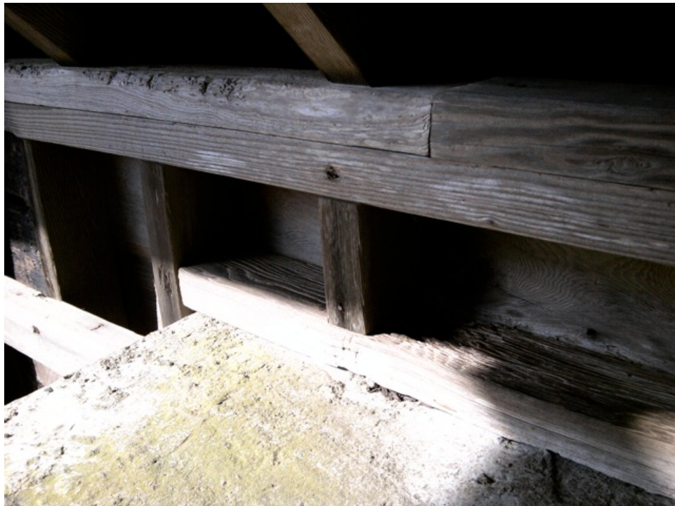
[Fig. 14] Detail of sill plate and roofing system, looking northwest.
