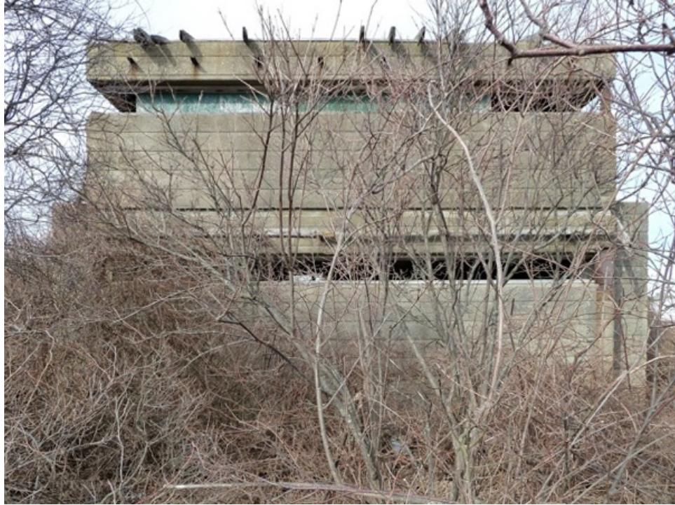
[Fig. 3] South elevation of Station 1-B, looking north. Note dense overgrowth.
