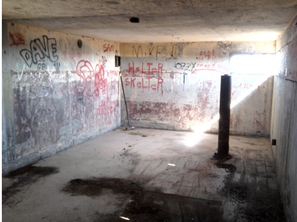
[Fig. 21] View of Room 2-1, looking southwest. Note original paint treatment.
