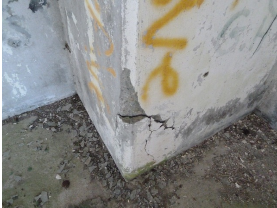
[Fig. 17] Detail of recessed southwest corner in Room 1-1, looking southwest.
