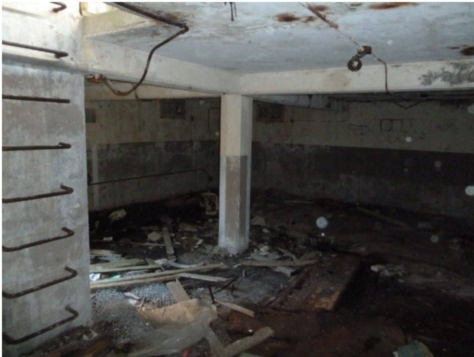
[Fig. 3] View of Room B-1, looking southeast. Note rust stains on the ceiling, debris, intact electrical conduits, and original paint treatment.
