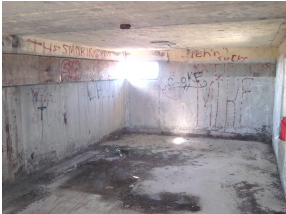
[Fig. 18] View of Room 2-1, looking southwest. Note original paint treatment.
