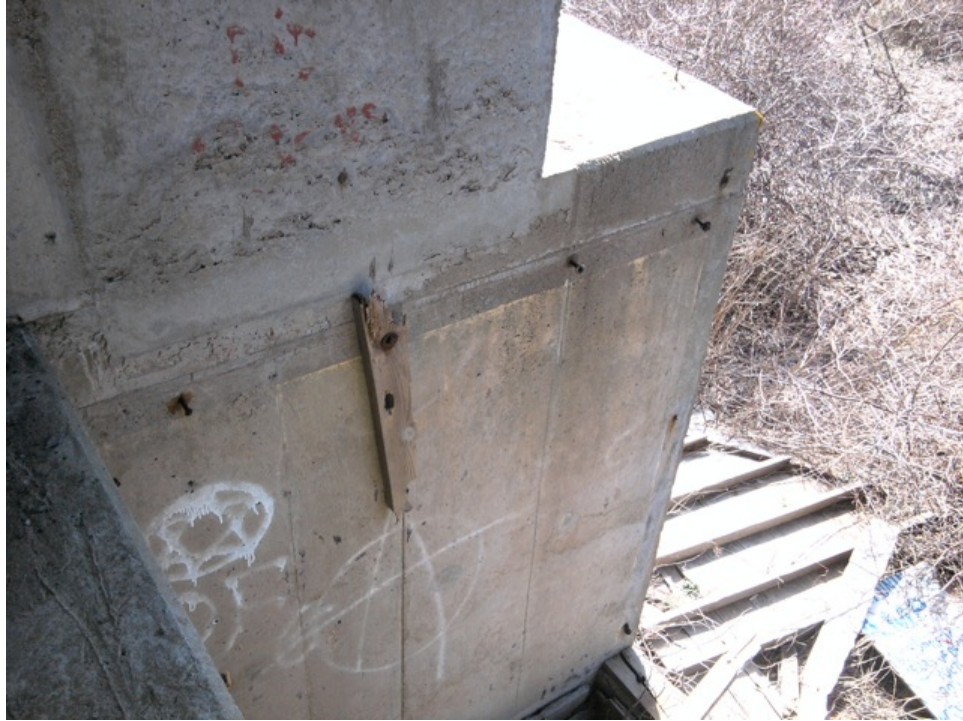
[Fig. 9] View of additional stair hall supports.
