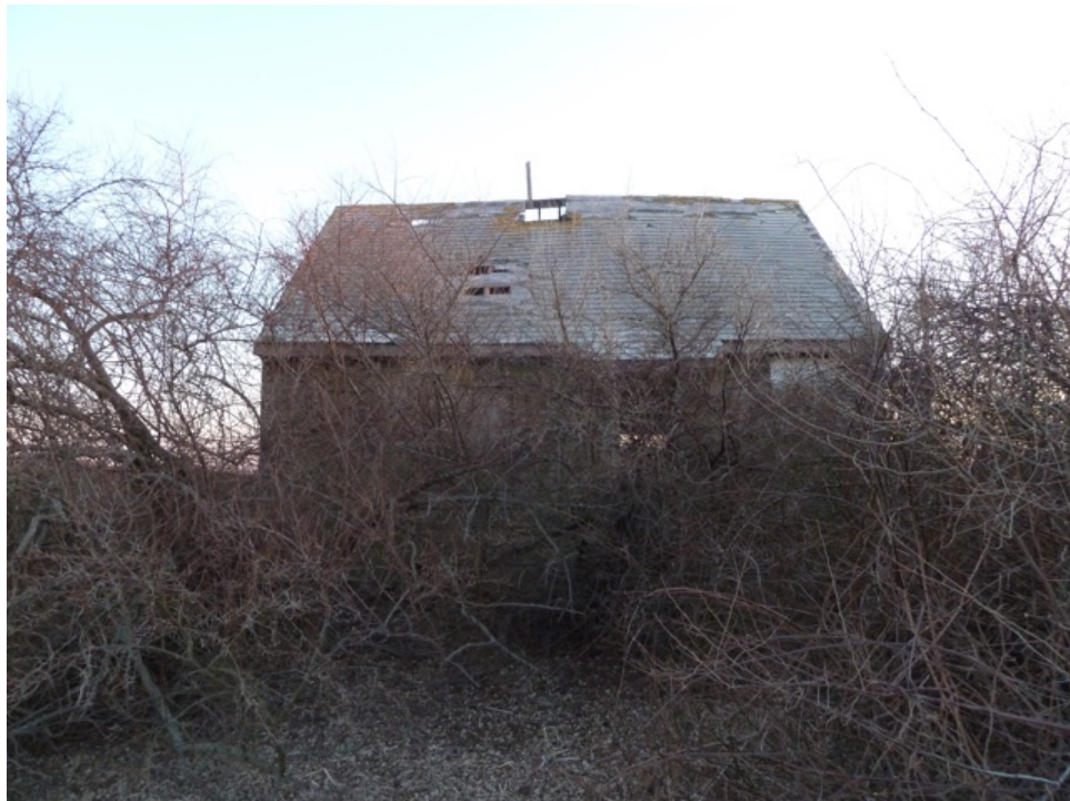
[Fig. 4] North elevation of Station 1-B, looking south. Note the scant remains of a false chimney.
