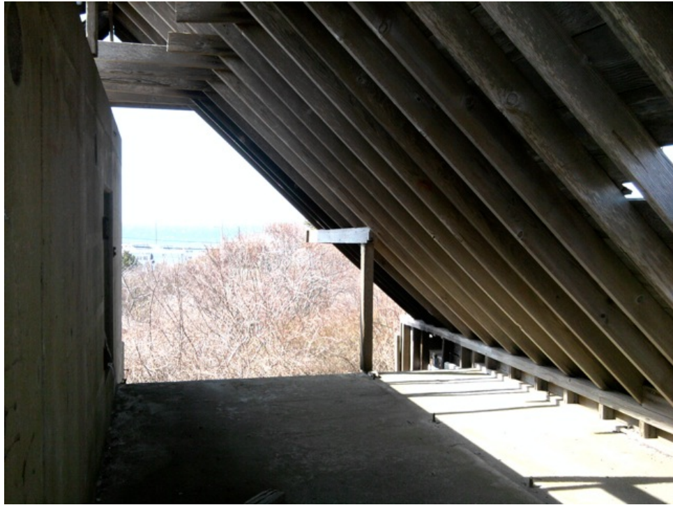
[Fig. 27] View of the east elevation of Room 2-2, looking west.
