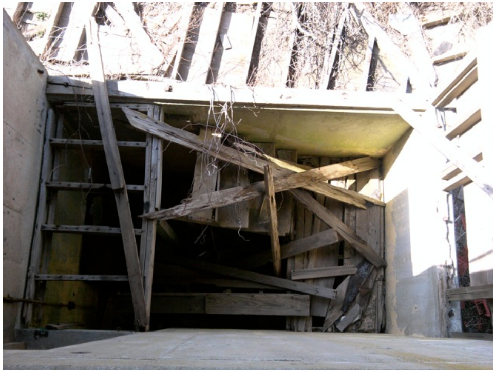
[Fig. 8] View of the stair hall from Room 2-2.
