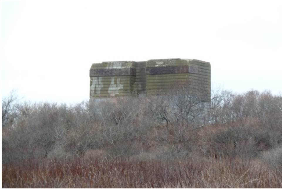
[Fig. 1] Southeast and northeast elevations of Station 3-A, looking west.
