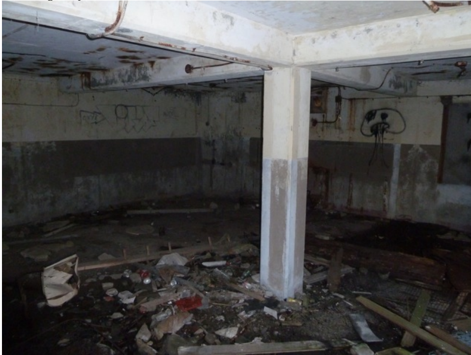
[Fig. 3] View of Room B-1, looking southeast. Note rust stains on the ceiling, debris, intact electrical conduits, and original paint treatment.
