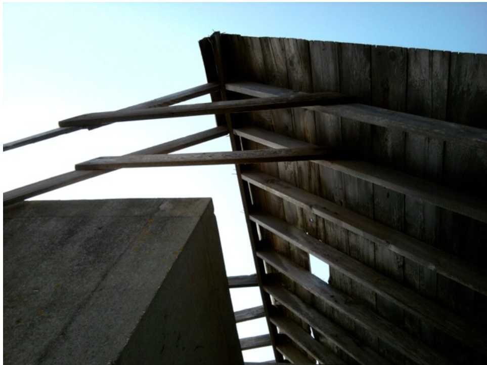
[Fig. 8] View of roof structure on the east elevation, looking west.
