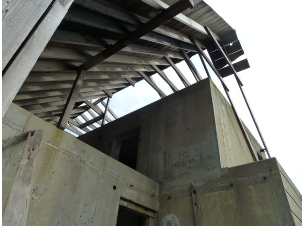
[Fig. 7] View of remaining roof structure and stair hall, looking southeast.
