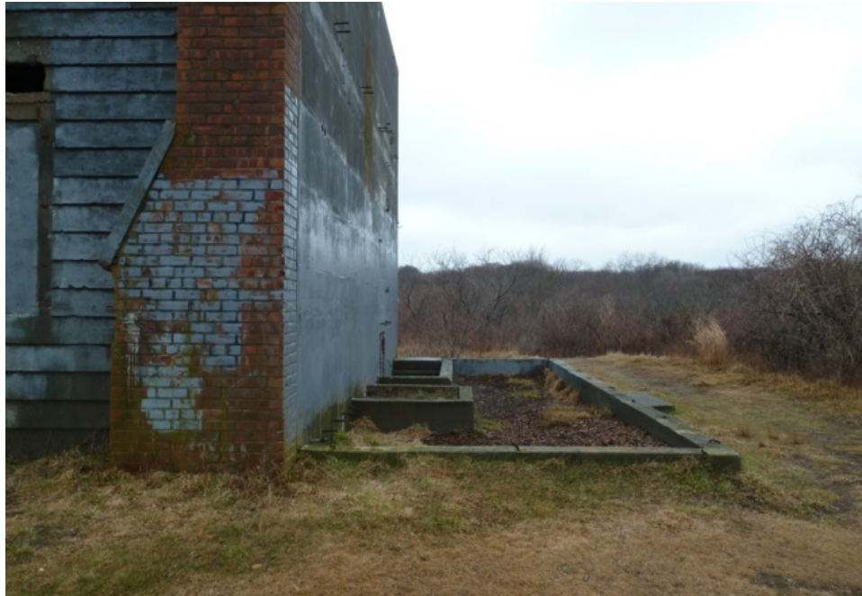
[Fig. 7] View of foundation, looking west.
