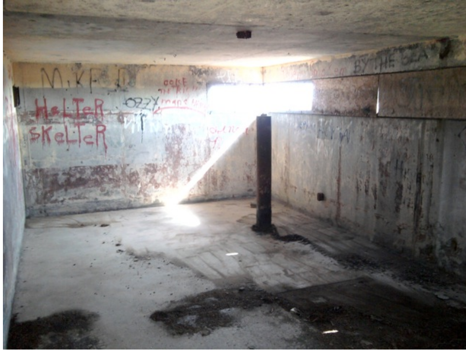
[Fig. 19] View of Room 2-1, looking southeast. Note original paint treatment and scope mount.
