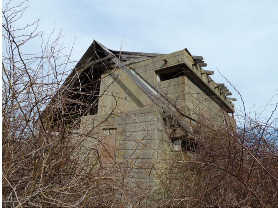
[Fig. 5] West and south elevations of Station 1-B, looking northeast.
