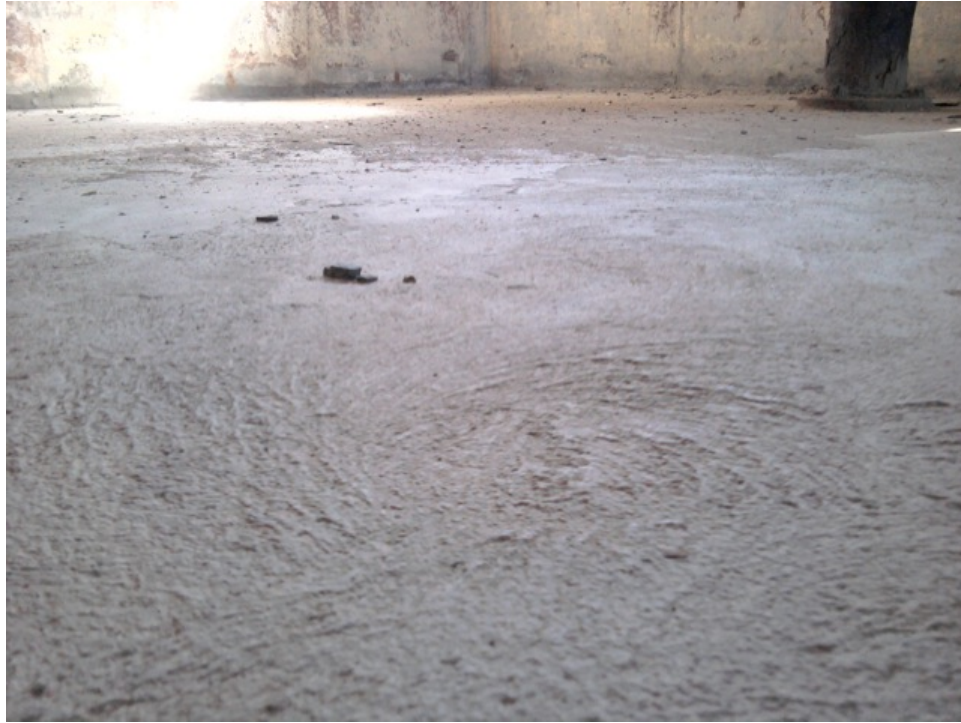
[Fig. 1] Detail of concrete floor in Room 2-1, looking southeast. Note the textured arc finish. The same pattern can also be found on the concrete floor in Rooms B-1 and 1-1.
