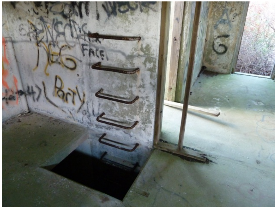
[Fig. 14] Detail of ladder rungs in Room 1-1, looking north.
