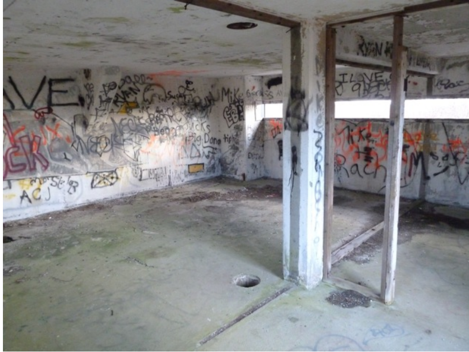
[Fig. 11] View of Room 1-1, looking southeast. Note the hole for a stove ductwork and original paint treatment under graffiti.
