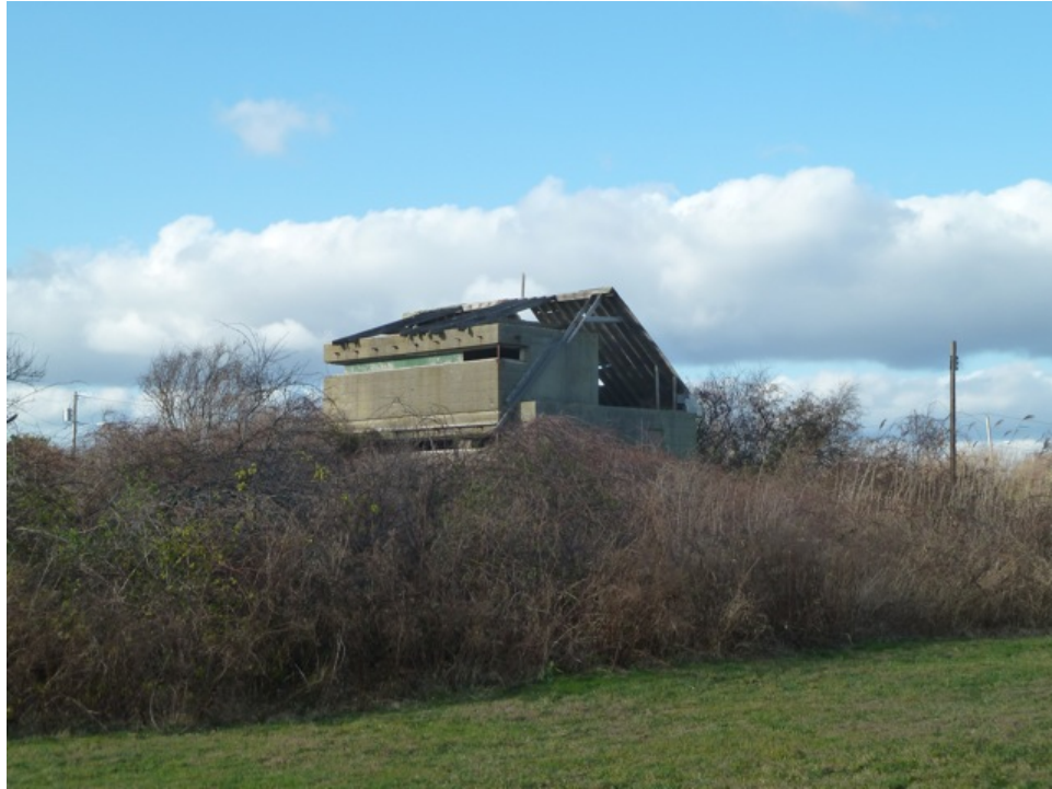
[Fig. 1] South and east elevations of Station 1-B, looking northwest.
