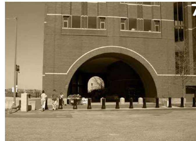
After crossing Northern Avenue you pass through the brick archway of the Federal Courthouse, which protects brilliantly viewed restaurant seating.
