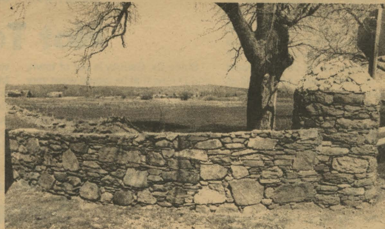
THE MAIN ENTRANCE, as it is seen today, was refurbished this spring in the same form as the original entrance looked like to Ferrycliffe Farm. MRS. FULTON has said that DR. FULTON was 'happy' with the recent reconstruction.
