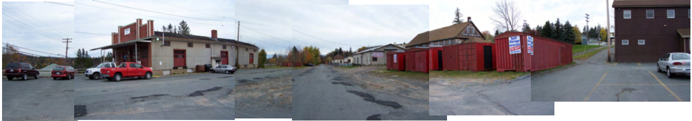
Existing Building to be used for Train Station
