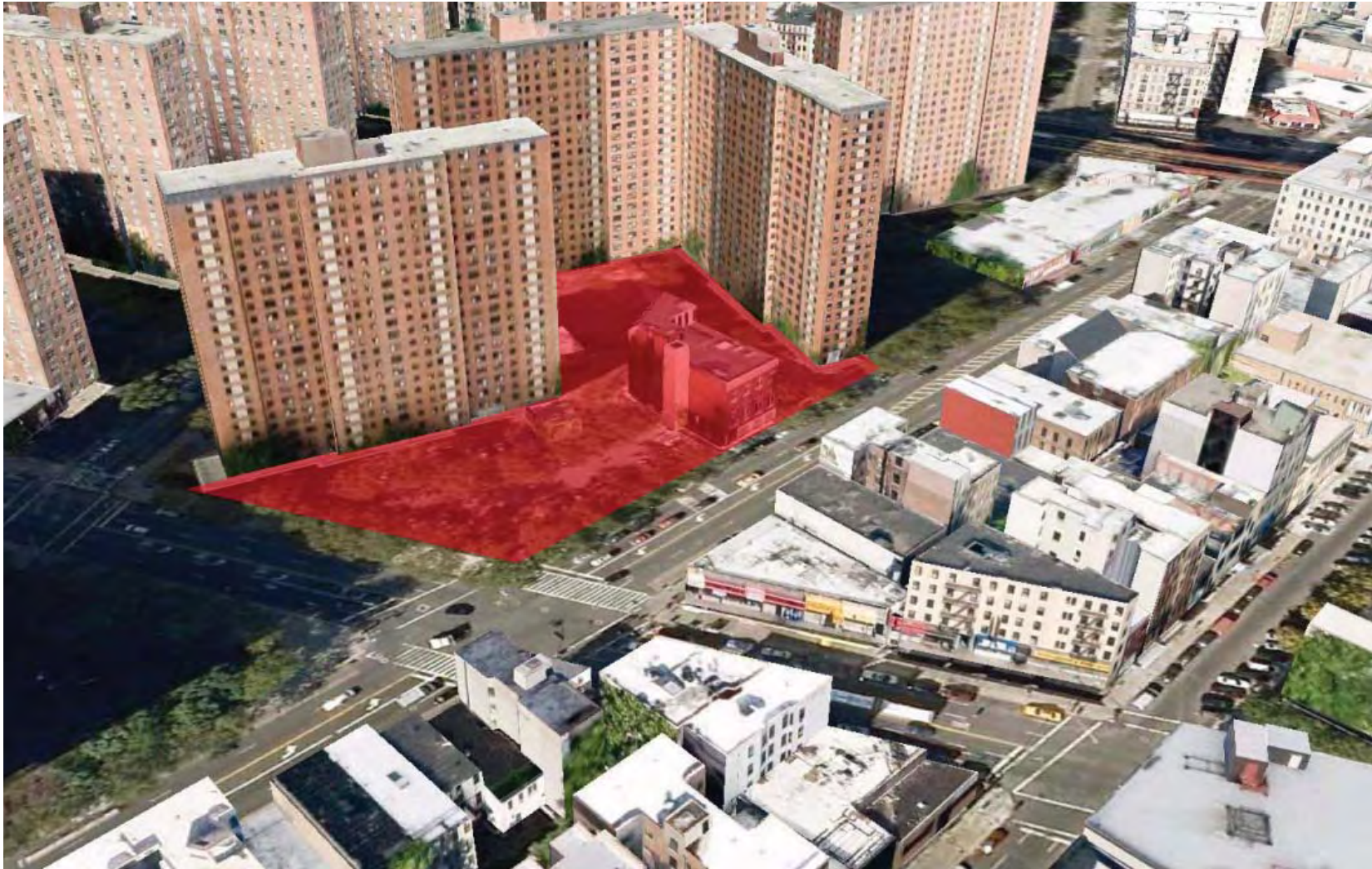
Site looking South-West
