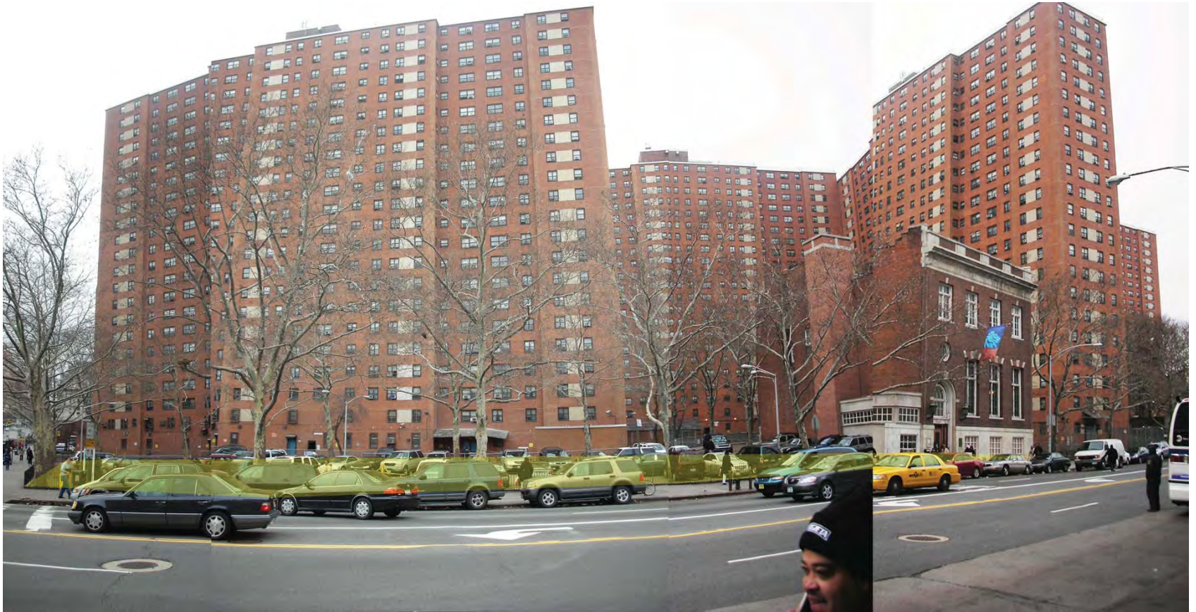
View from across the street looking south at the site
