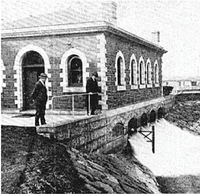
Figure 54: Troy Street Pump Station
