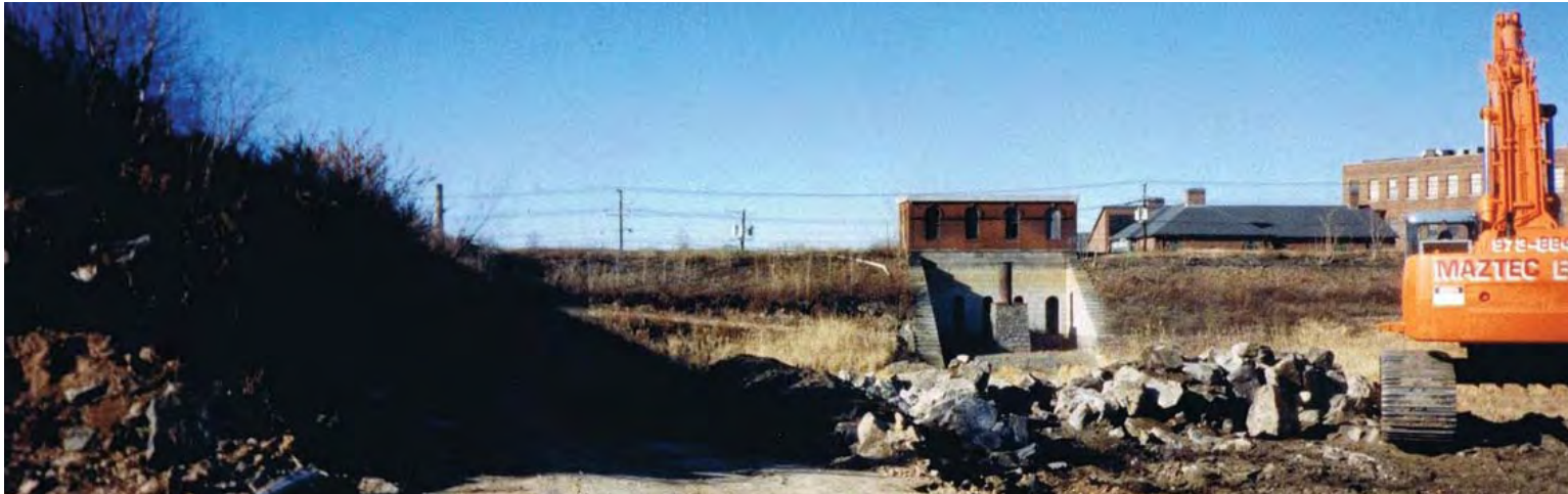
Figure 25: Decommission and Excavation of the Reservoir
