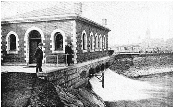
Figure 21: Troy Street Pump Station
