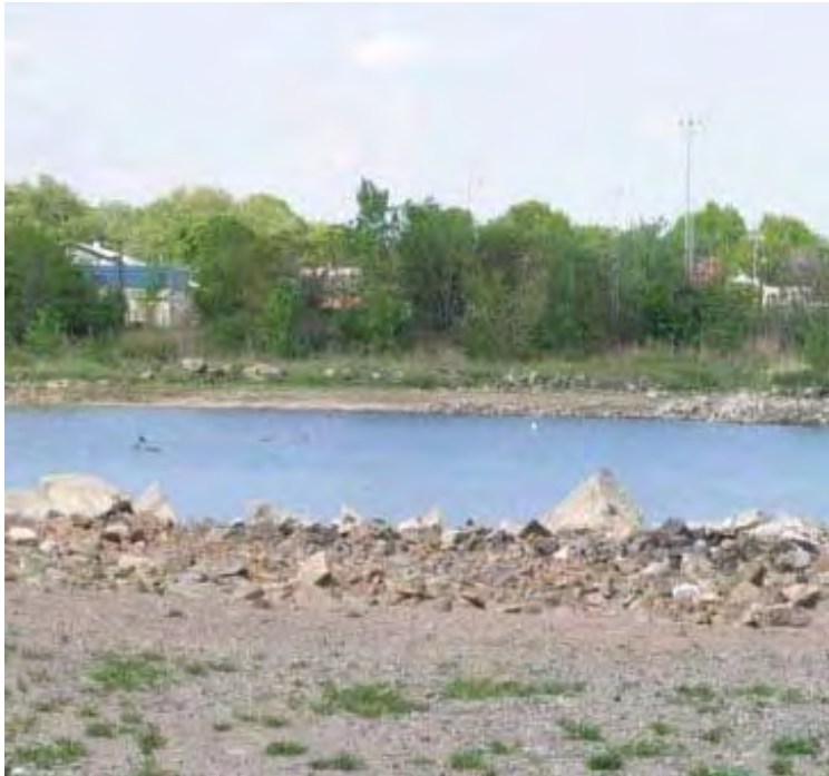
Figure 28: Image of the Reservoir
