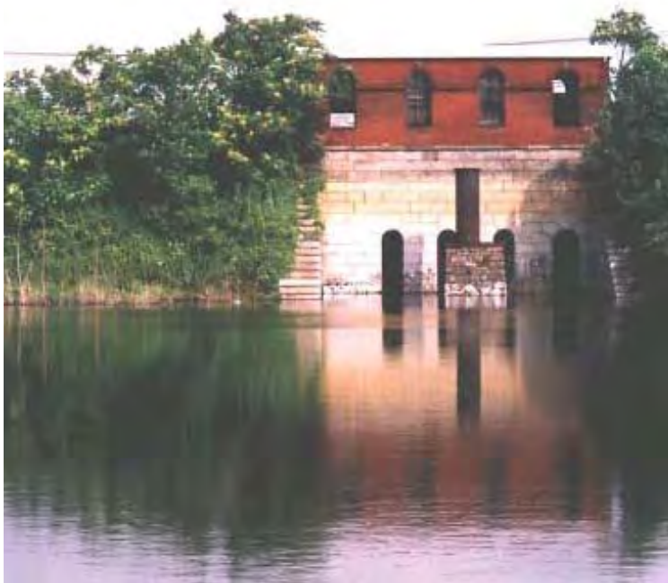
Figure 30: The Pumping Station
