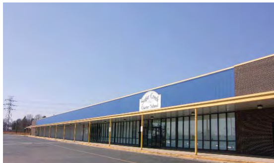
Charter School Renovated K-Mart
