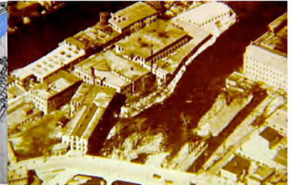
Image 44 WOONOSCKET VILLAGE- TRENCHES & CANALS 1938
