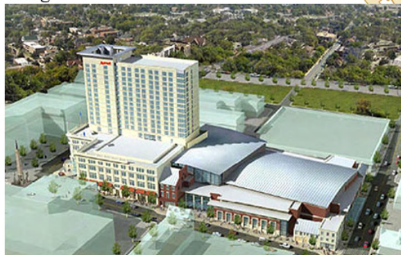
Lancaster County Convention Center
