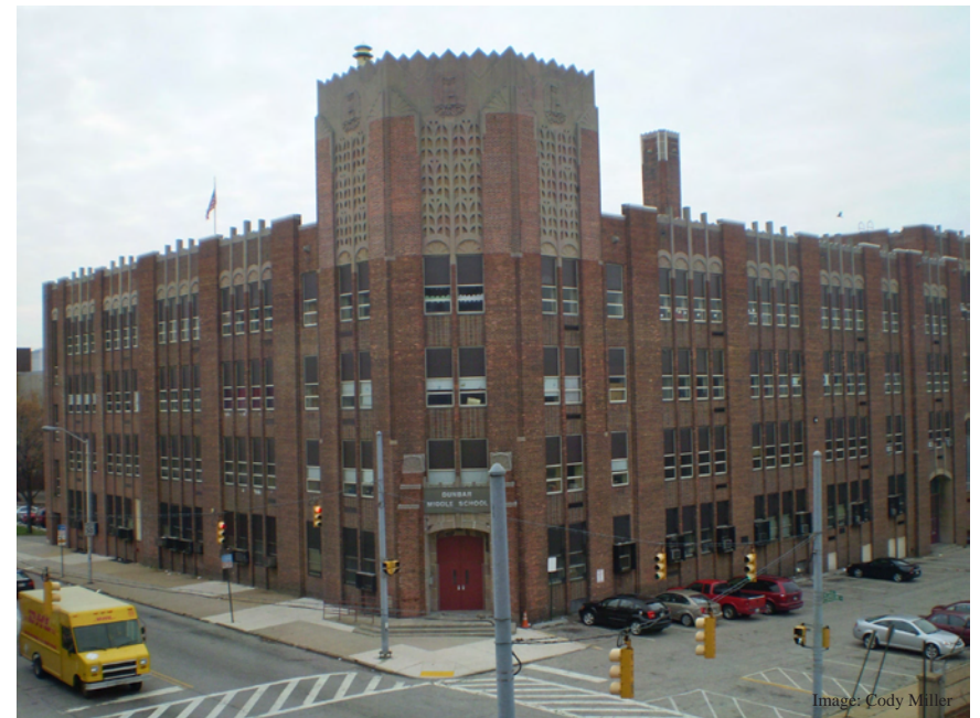
Dunbar Middle School is located on the sites adjacent city block
