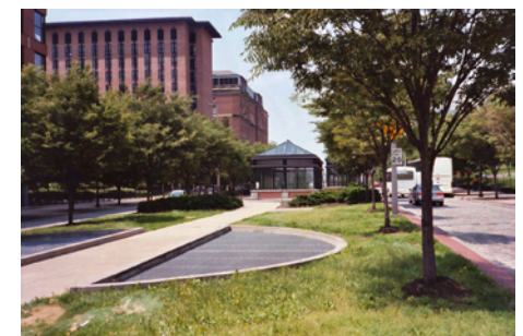
View of metro station access looking north
