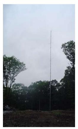
As part of the wind feasibility study, Weston & Sampson erected a 50-meter tall Meteorological tower (MET tower) for monitoring wind, and is currently preparing a wind feasibility study in accordance with MTC requirements.
