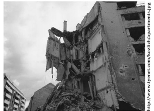
Apartment Building in Ruin
