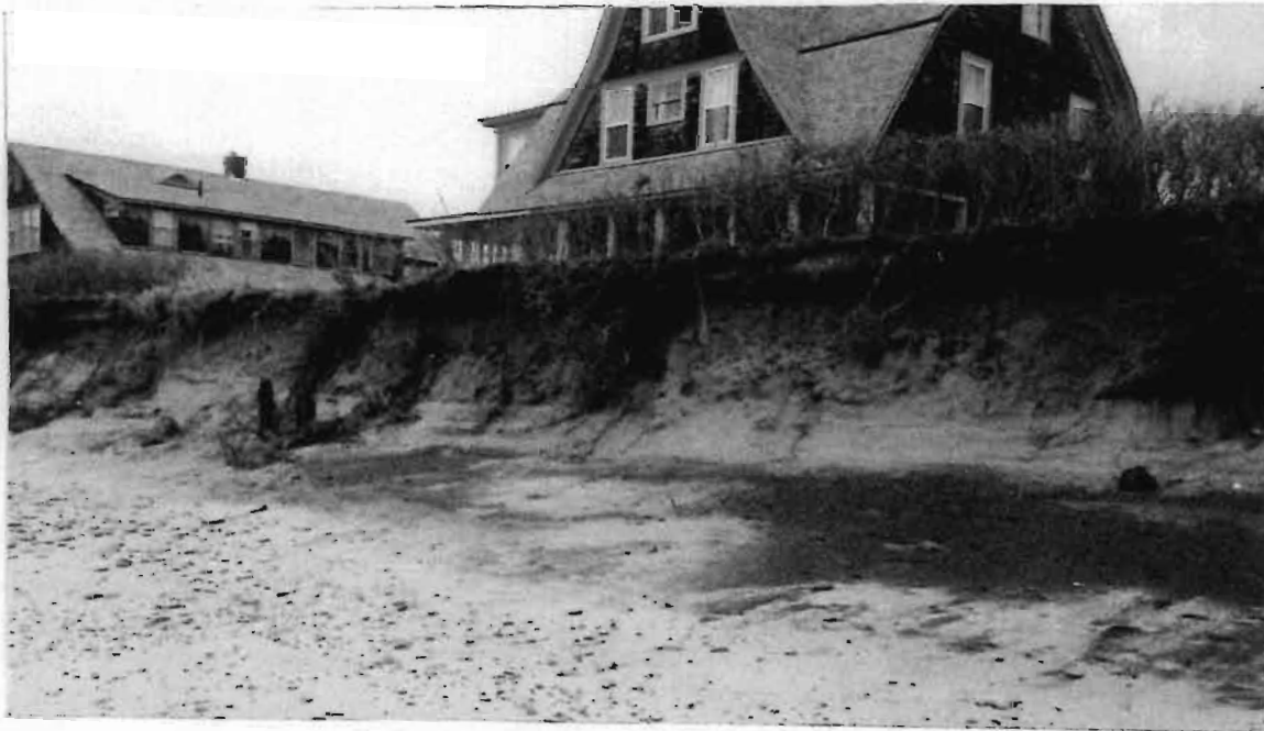
RIGHT TO LEFT HARRIS AND DUVAL COTTAGES MARCH 1991
