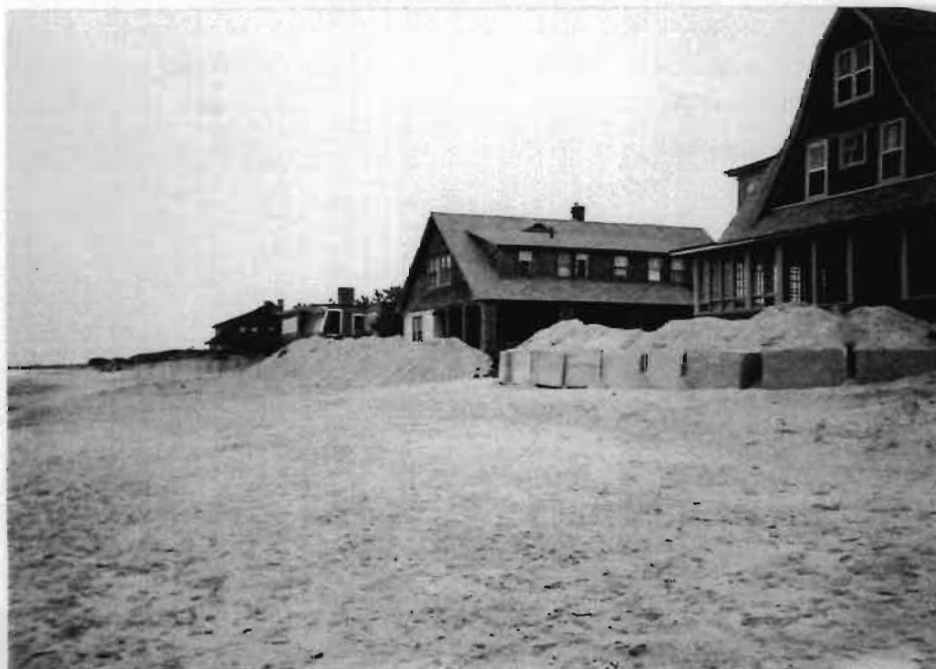
HARRIS, DUVAL, CHAFFEE AND WESTERN MOST COTTAGE VIEW TO WEST NOVEMBER 1991
