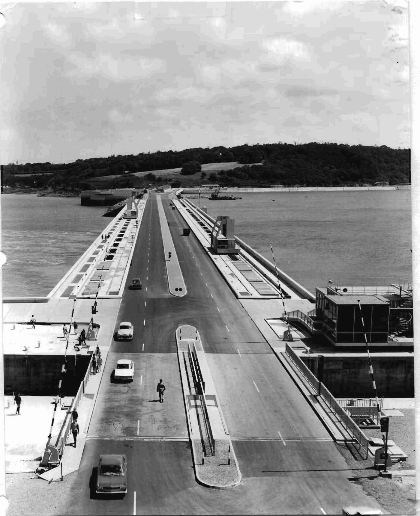
FIGURE 10. RANCE RIVER POWER PLANT
