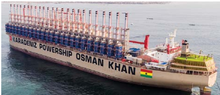
Figure 7.13: The Osman Khan, one of the Turkish generator ships which has been temporarily relieving Ghana's power crisis since 2015.
