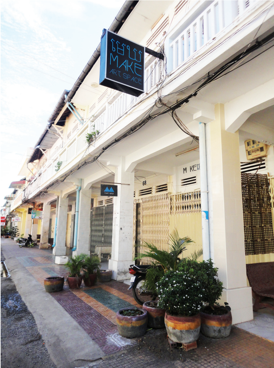
Figure 38: Gallery Maek Make, Battambang (2014). Source: personal documentation.
