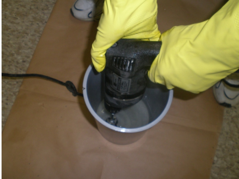
Figure 3.16: Mixing of epoxy components
