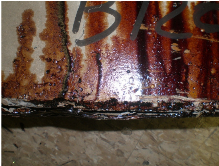
Figure 6.143: FRP delamination of B120-180°C, 100% RH
