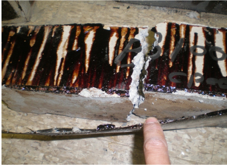
Figure 6.123: FRP delamination of concrete beam specimen, 180°C and 250 cycles
