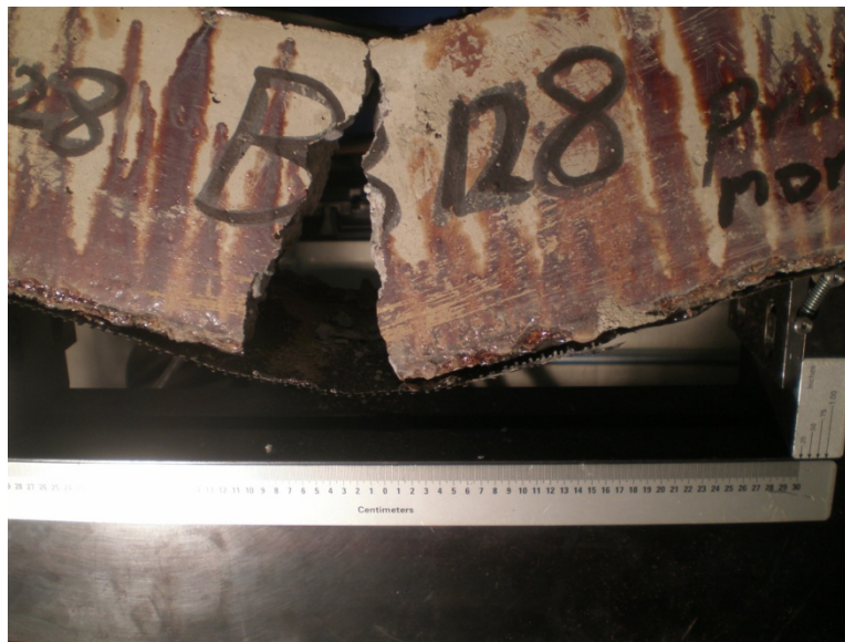
Figure 8.10: Concrete flexural crack and FRP delamination, B128
