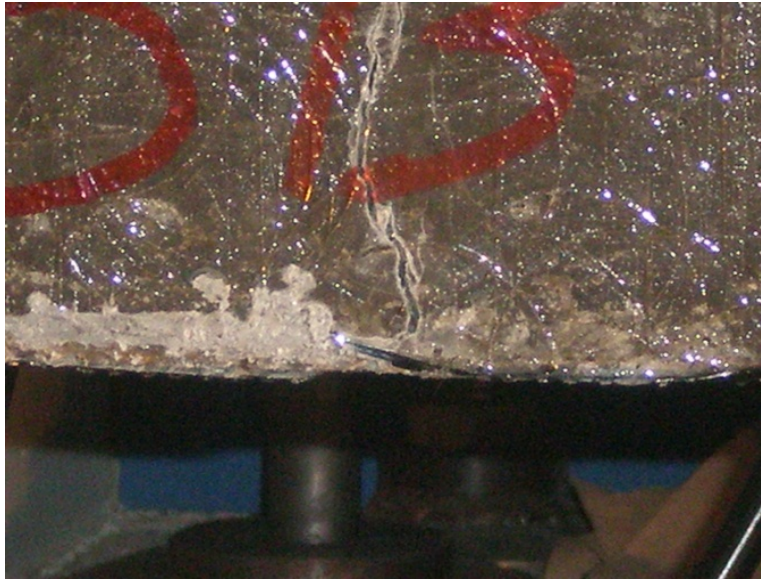
a) Concrete flexural crack, B13
