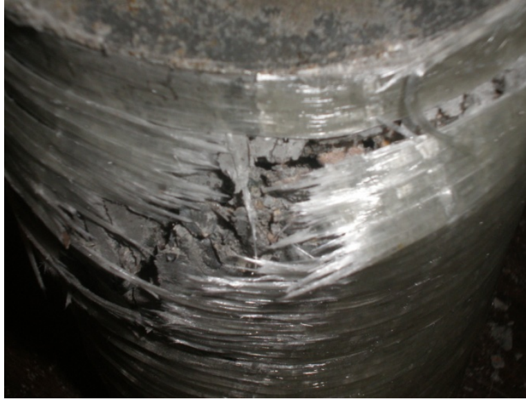
a) Concrete crushing and GFRP rupture of C4T1
