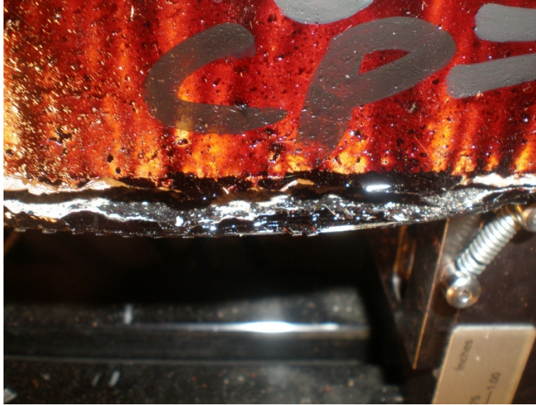
Figure 6.121: FRP delamination of concrete beam specimen, 180°C and 100 cycles
