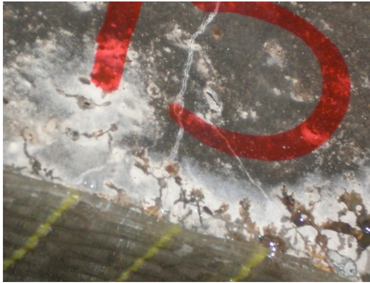
a) Concrete flexural crack followed by shear crack of specimen B15
