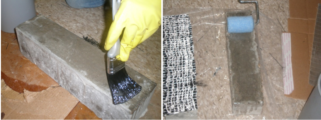
Figure 3.17: Applying epoxy on beam concrete surface
