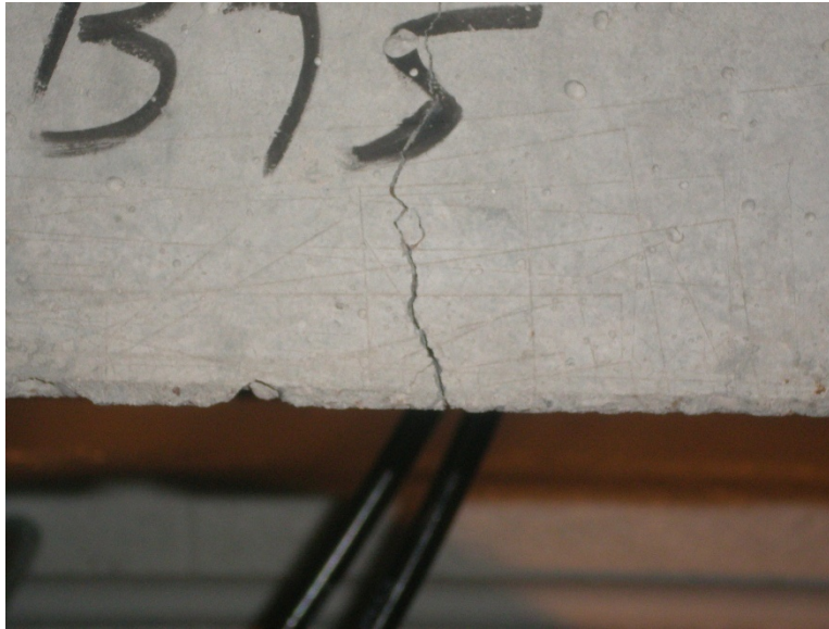
Figure 6.9: Flexural failure of concrete beam-180°C
