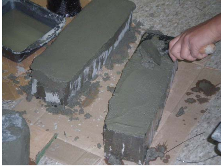
Figure 8.2: Protection of FRP sheets with cement mortar
