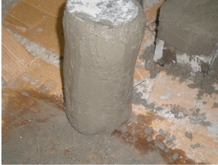
Figure 8.6: Strengthened columns protected by cement mortar
