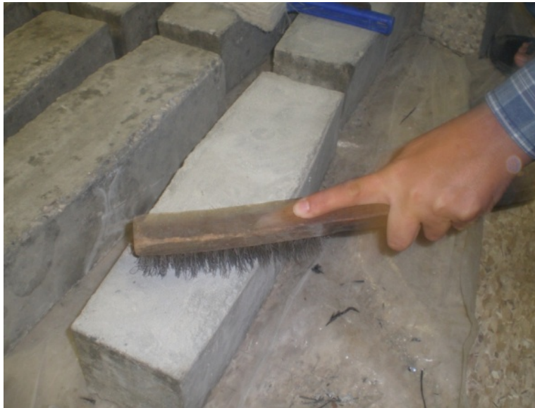
Figure 3.15: Concrete surface cleaning
