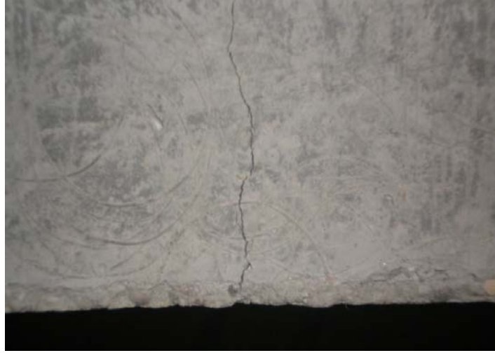
Figure 6.3: flexural failure of control concrete beam B2
