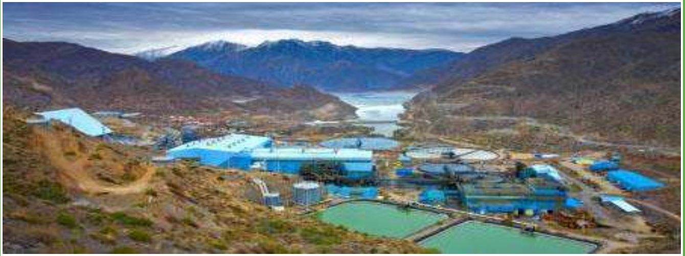
Los Pelambres Mine, panoramic view of the concentrated copper process Source: Bechtel Corporation ( www.bechtel.com/los-pelambres-mine.html )
