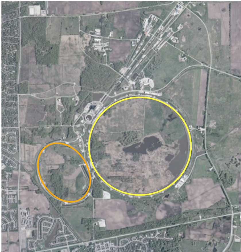
Figure 4.1: Aerial view of the FNAL accelerator complex. The Tevatron (yellow highlight) is the large circular (radius of 1 km) object in the center of the photo. The main injector (orange highlight) is also shown.
