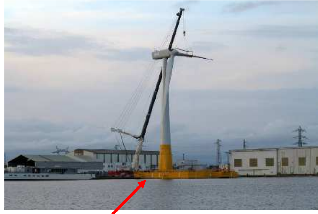
Crane for outfitting
