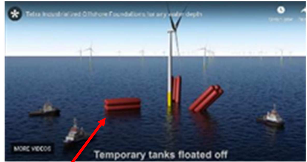
Remove temporary buoyancy after Connecting tendons
