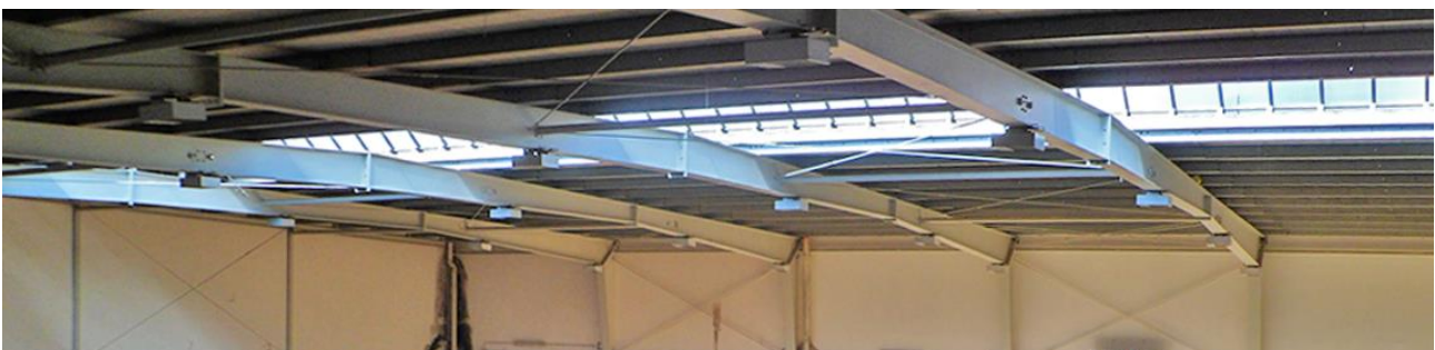
Figure 3. 31: particular of the roof of the sport palace
