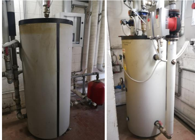
Figure 3. 13: water storage tanks on the cold (on the left) and hot side (on the right) of the heat pump
