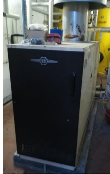
Figure 3. 3: gas burners used to integrate DHW/SH needs in the heating system of the Palacus sport palace. a) burner for only DHW out of the heating season – 35 kW peak thermal power; b) burner for DHW and SH during the heating season – 320 kW peak thermal power
