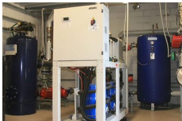
Figure 2. 4: solar assisted heat pump with bare solar thermal panels – Sestri Levante (GE) – (22)
