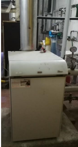
Figure 3. 3: gas burners used to integrate DHW/SH needs in the heating system of the Palacus sport palace. a) burner for only DHW out of the heating season – 35 kW peak thermal power; b) burner for DHW and SH during the heating season – 320 kW peak thermal power
