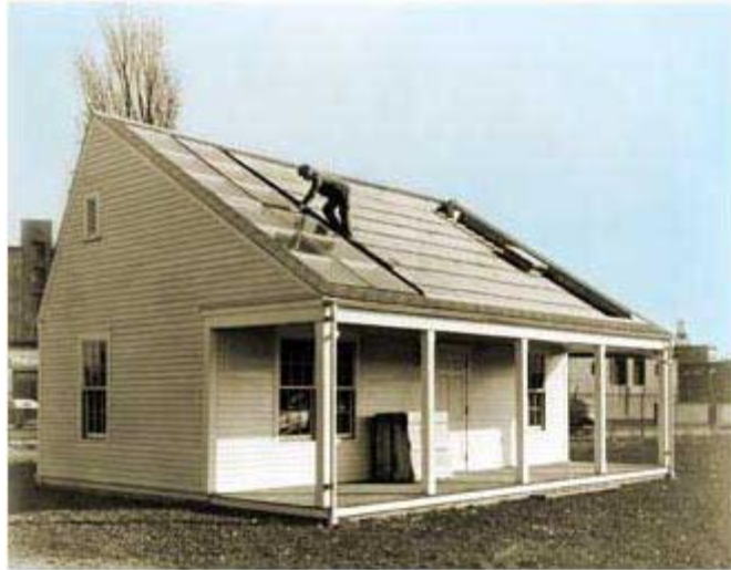
Figure 2. 13: solar house built by MIT, in 1939, (52)
