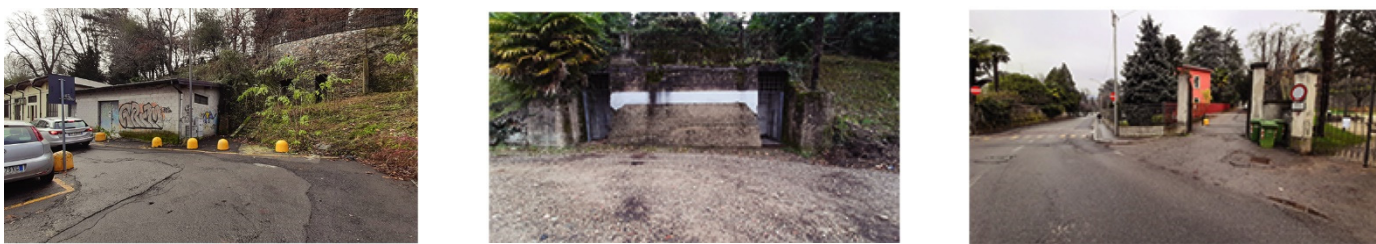
Figure 5. Views of the various entrances to the bunker. Photos by A. Pilo.
