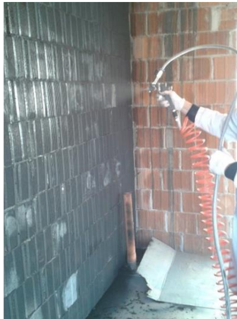
Figure 6. Application by spray of SUNSPACE on a wall of a structure of the Department of Civil Engineering of the University of Brescia [58].
