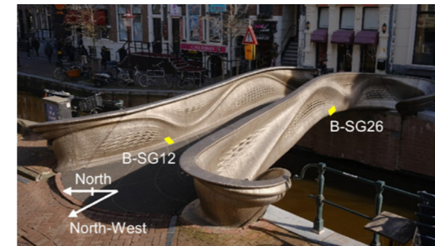
Fig 1 The MX3D Bridge in Amsterdam
