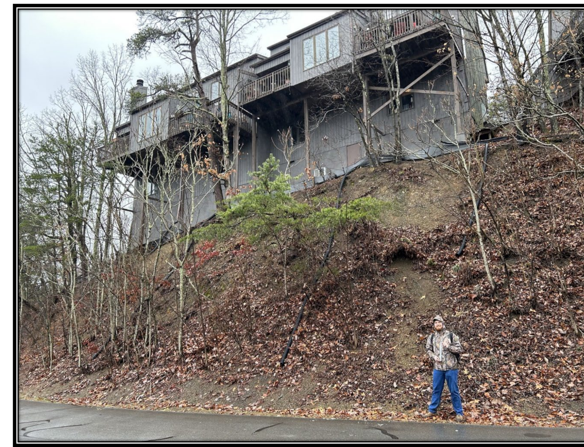
Figure 4: A picture of a steep slope behind some of the houses, the slope here was 51°.
