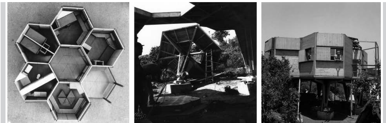
Figure 1. (left) The model of Casa Esagono and (center and right) the house under construction [source: B.A.Co Vittorio Giorgini Archive]
