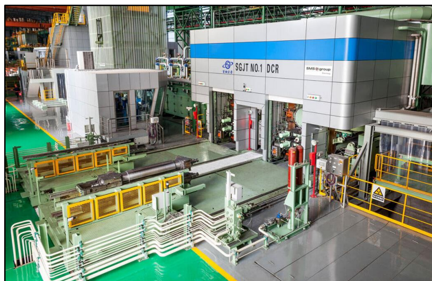
Figure 4: Shougang Jingtang United Iron Steel Co. Ltd Facility, Tangshan China
